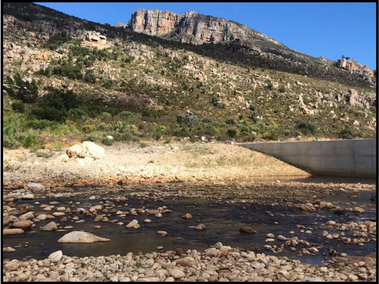
FIGURE 5: UPSTREAM OF WEIR; LEFT EMBANKMENT.
