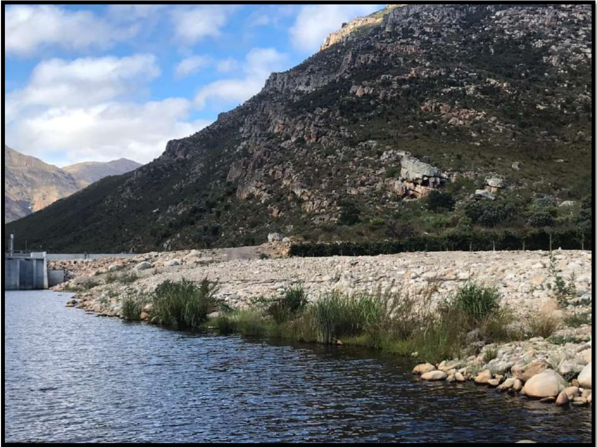
FIGURE 7 DOWNSTREAM OF WEIR; LEFT EMBANKMENT.
