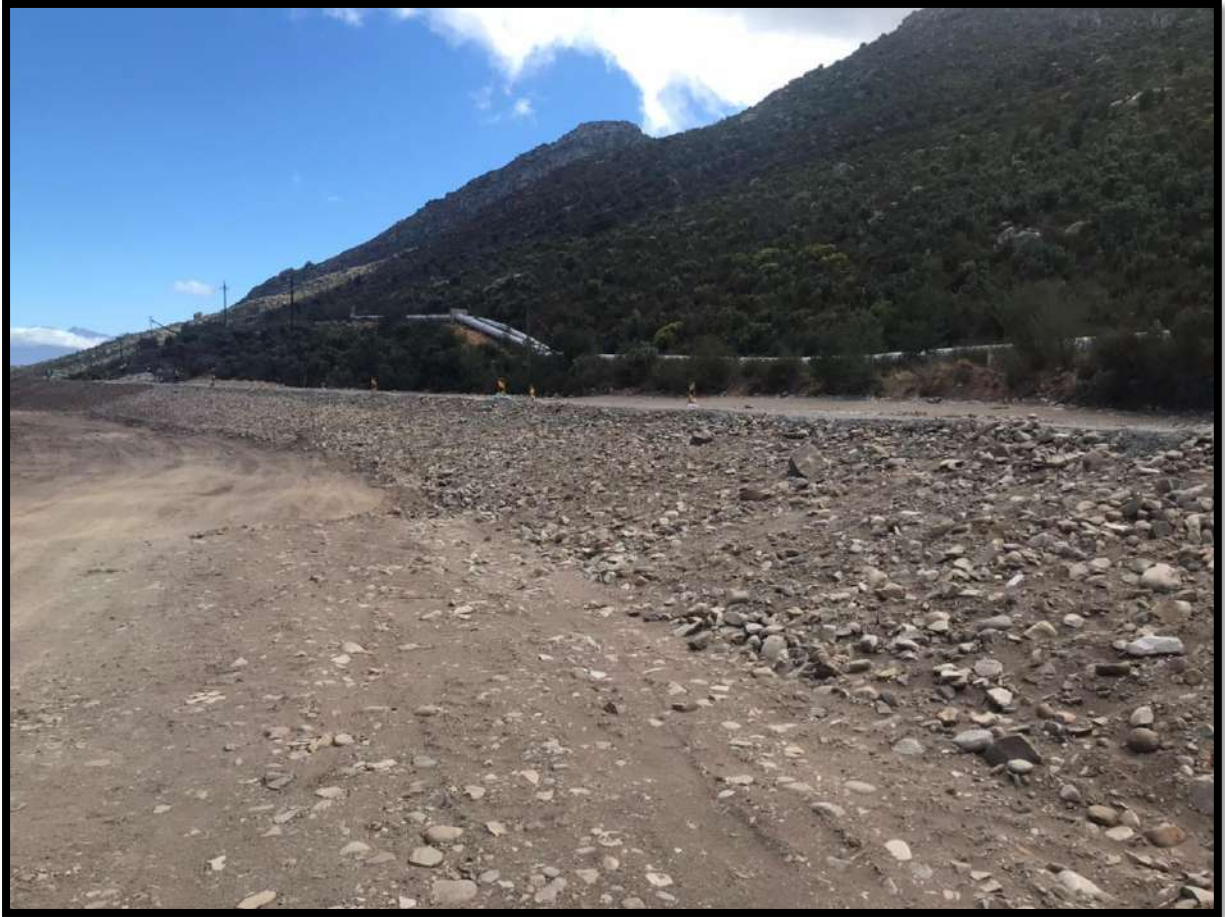
FIGURE 4: EMBANKMENT ALONG STETTYNS ROAD.
