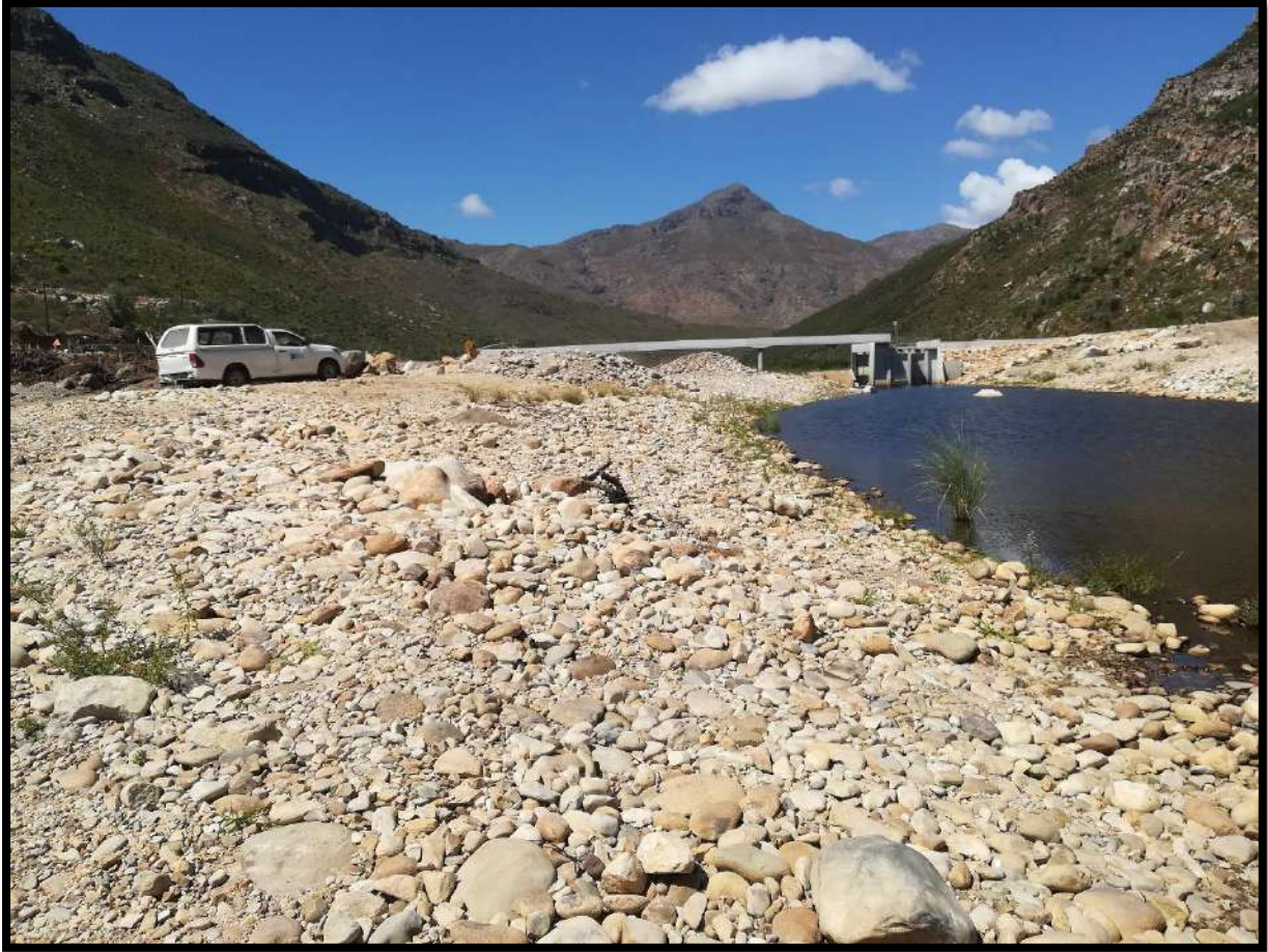
FIGURE 6: DOWNSTREAM OF WEIR; RIGHT EMBANKMENT.
