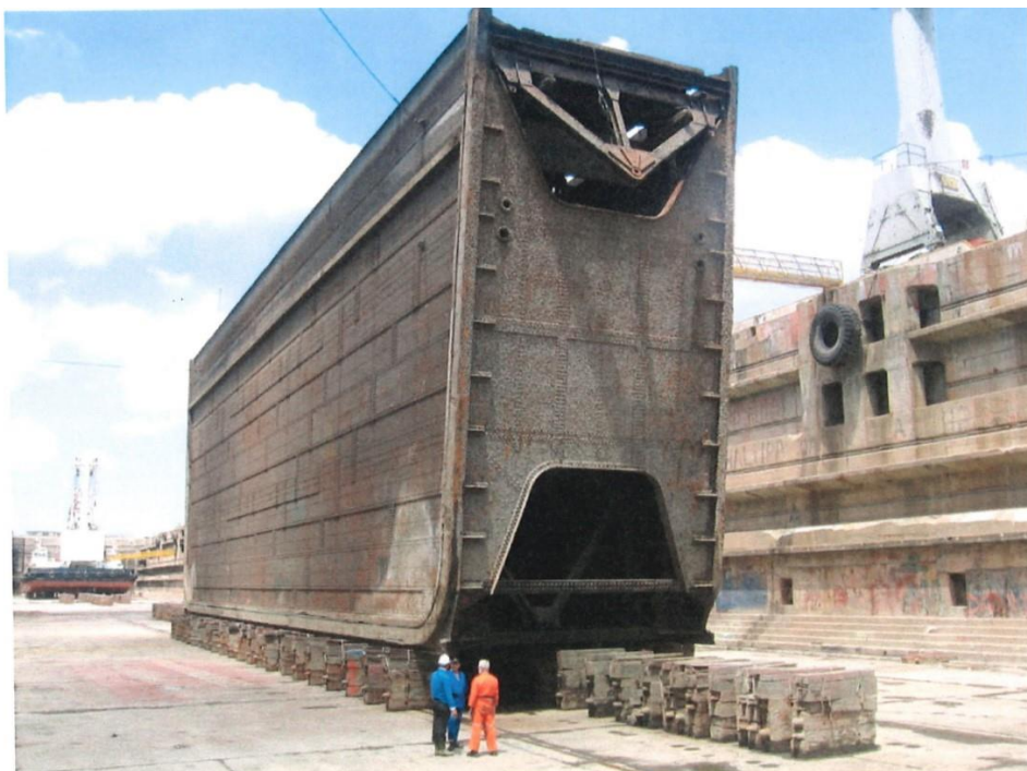
Figure 5: Sturrock Dry Dock Sliding Caisson Gates (in Dock)
