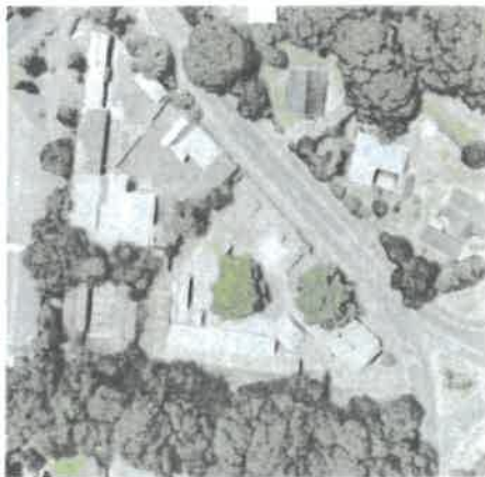
Site Aerial View
