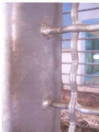
Mesh welding to frame (terminal)
