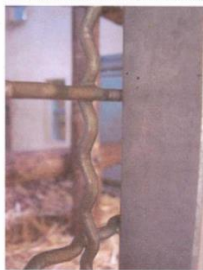
Mesh welding to frame (intermediary)
