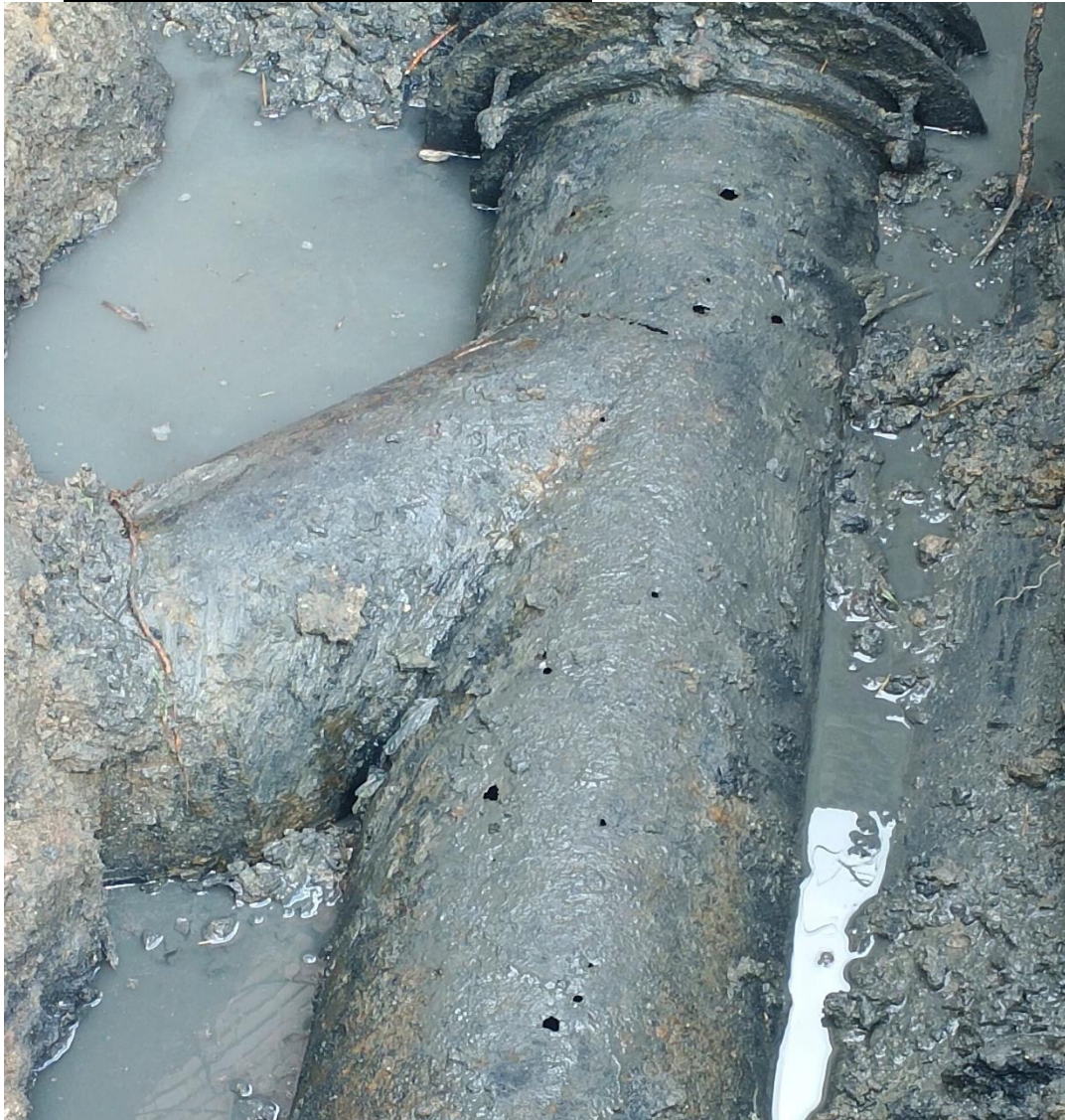
Fig. A. Existing pipe to be replaced
