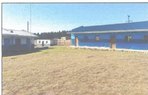
Picture 1: Looking approximately east towards the main school buildings.
