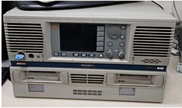
Racal Wordnet Series 2 Voice recorder/logger, Location: PABX Room K1
