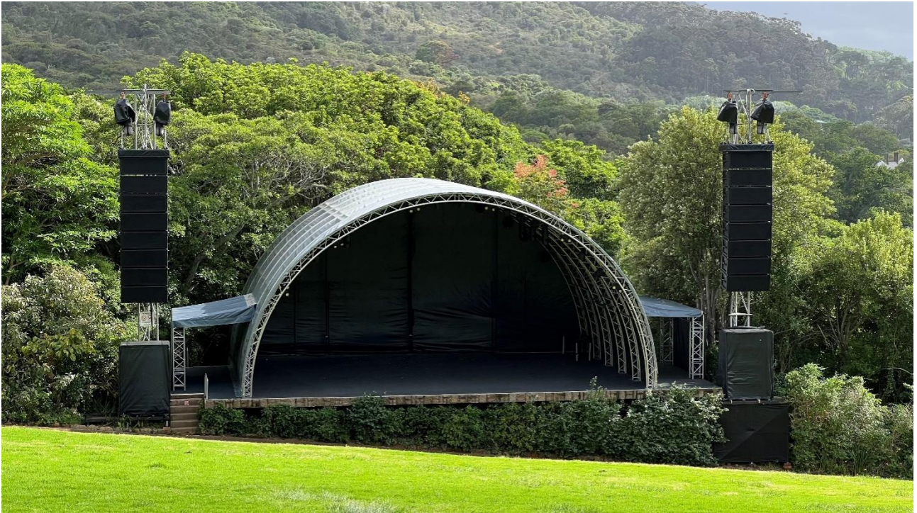
Figure 3. Tunnel concert stage canopy with “cowsheds” on either side.
