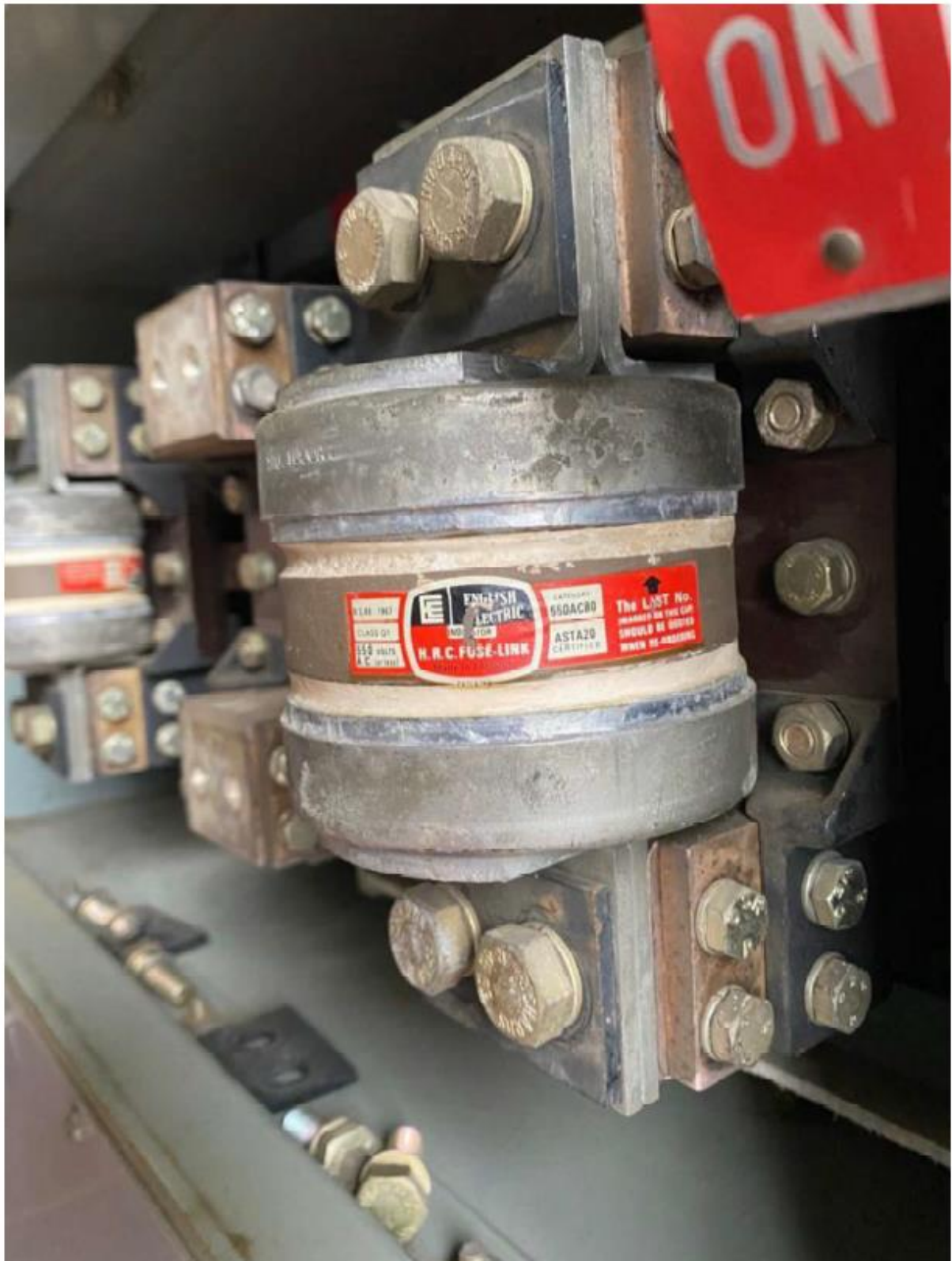
Picture: 550V AC / 1000A fuse link
