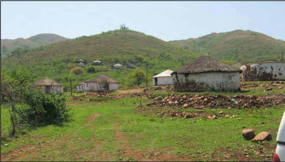
Picture 13: Current housing is in small clusters, many on small cut and fill platforms.
