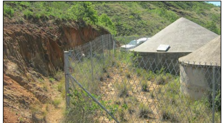
Picture 39: Reservoir and Pump-Room 3-10
