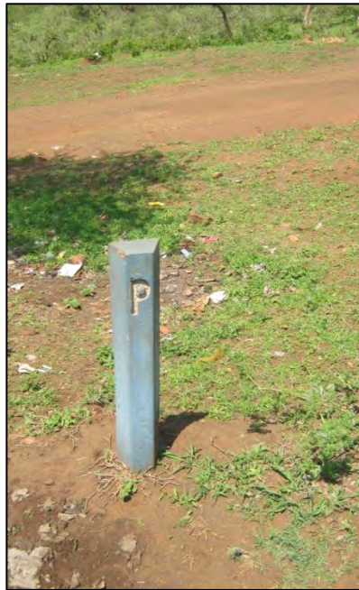
Picture 33: Pipe markers noted on site.
