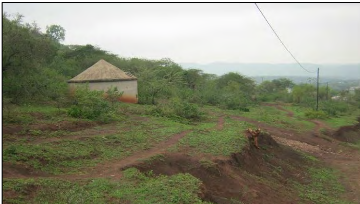
Picture 38: Reservoir and Pump-Room 3-6
