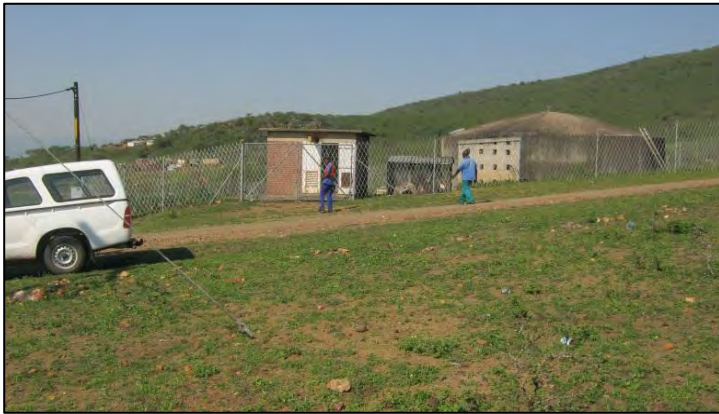
Picture 36: Reservoir and Pump-Room 3-1
