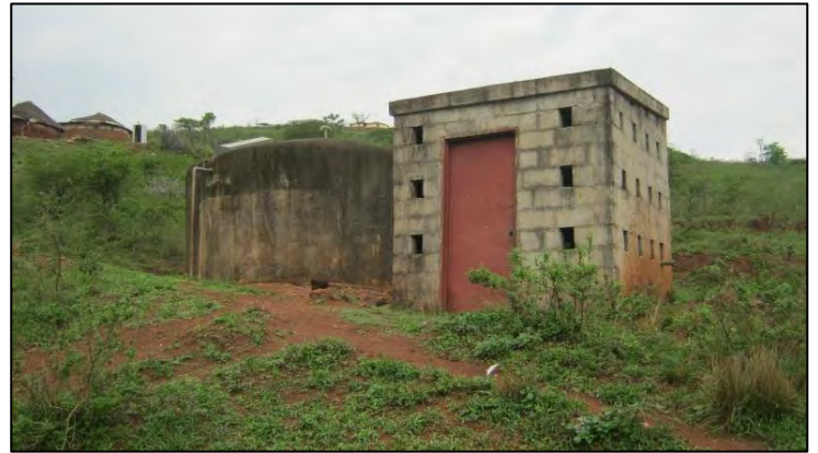
Picture 37: Reservoir and Pump-Room 3-2
