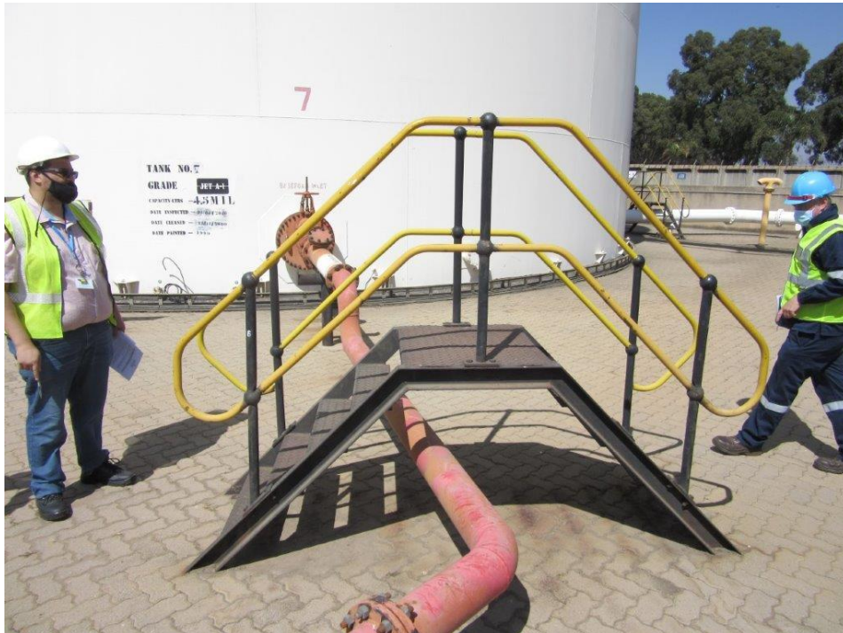
Figure 1: Bridged over-pipe walkway
