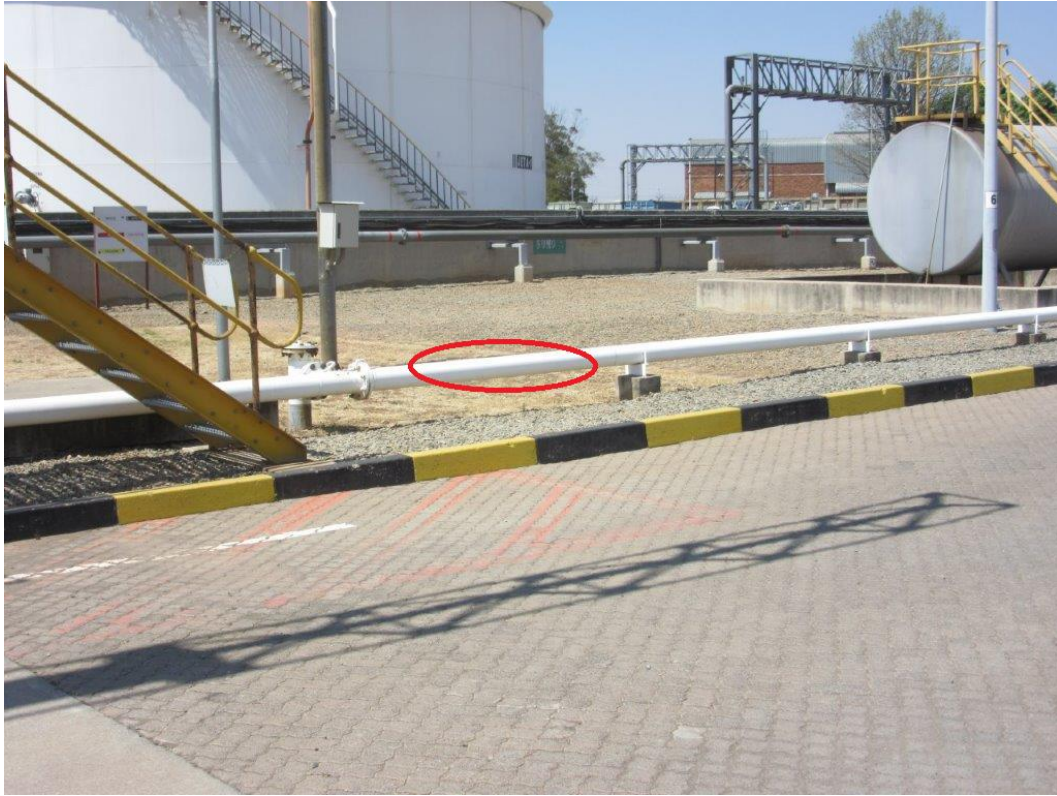
Figure 7: Small-sized bridged walkway
