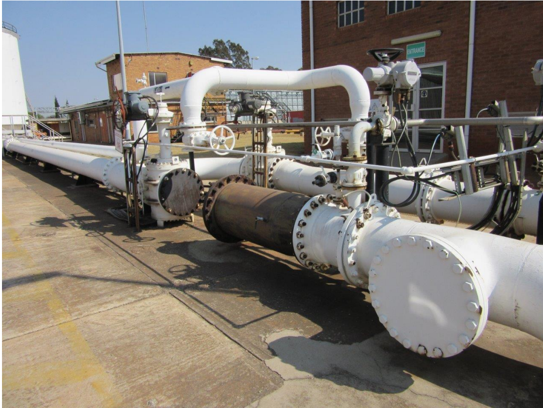
Figure 4: D1 and D2 actuated valves (D2 de-commissioned) reverse angle
