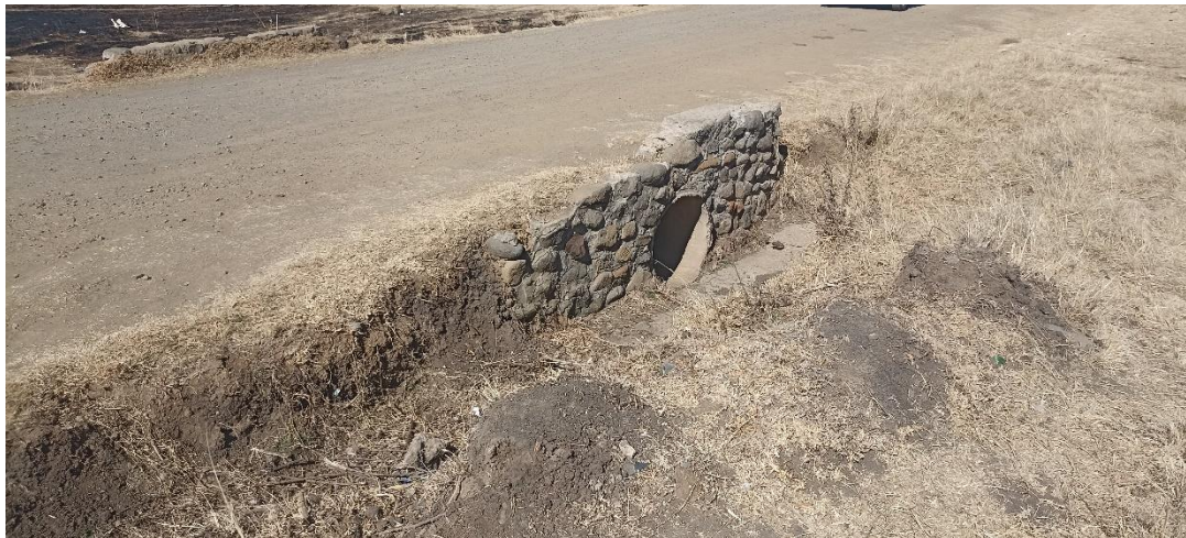
Existing Stormwater concrete pipe inlet
