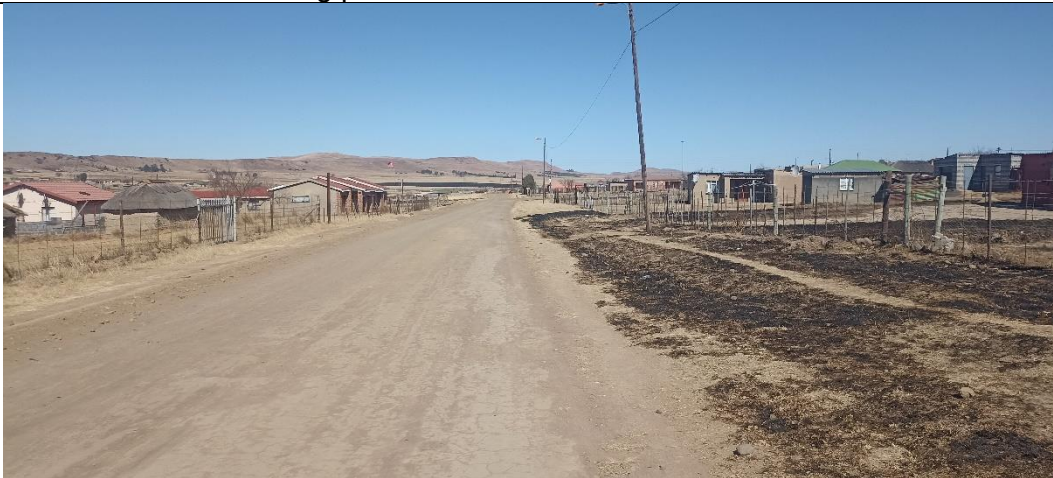
Existing Gravel Road
