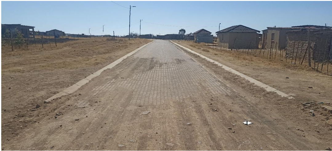
Start of Road with existing paved road
