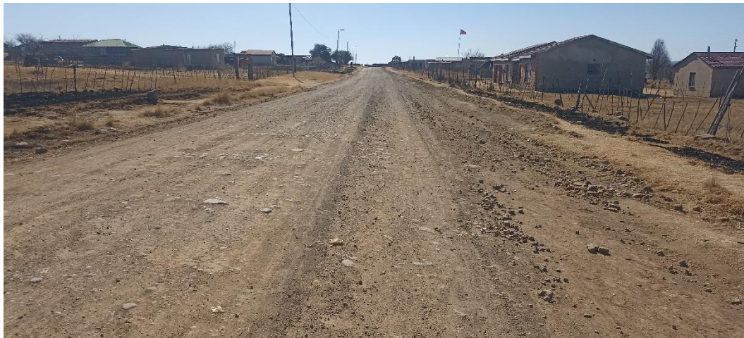
Existing gravel road
