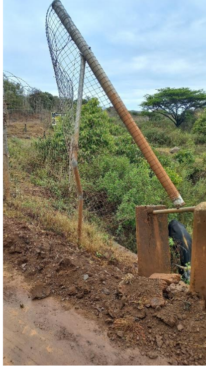
End of fencing repair on left bank. Total repair =57m on right bank, includes new fencing, y-standards, foundation and poles.
