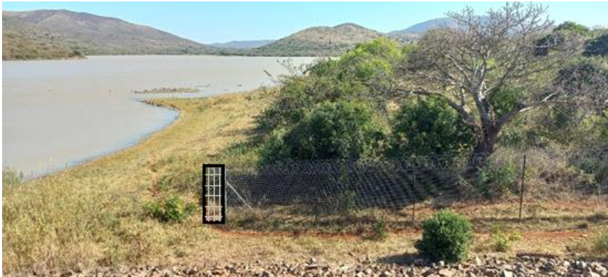
Dam wall left bank easily accessible by livestock and community
