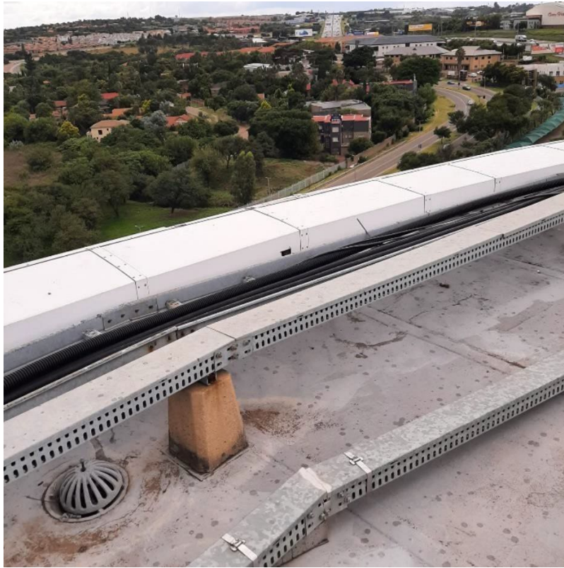
View from the top of the building indicating Sector 1
