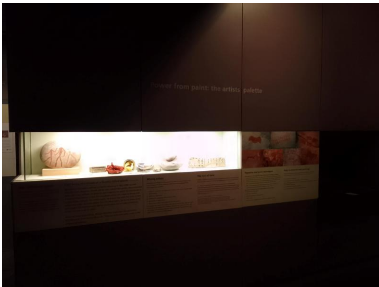
Figures 5. Demolish display cases and restoration of walls. Wooden Panels to removed behind display cases.
