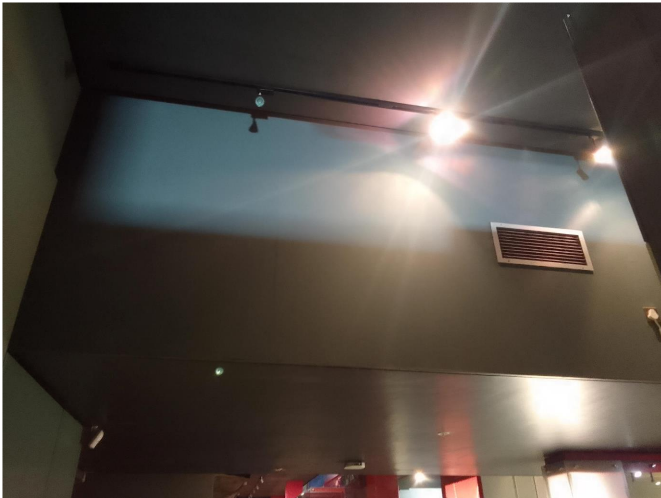
Figures 4. Adjust current ceiling to certain height and restoration of original ceiling
