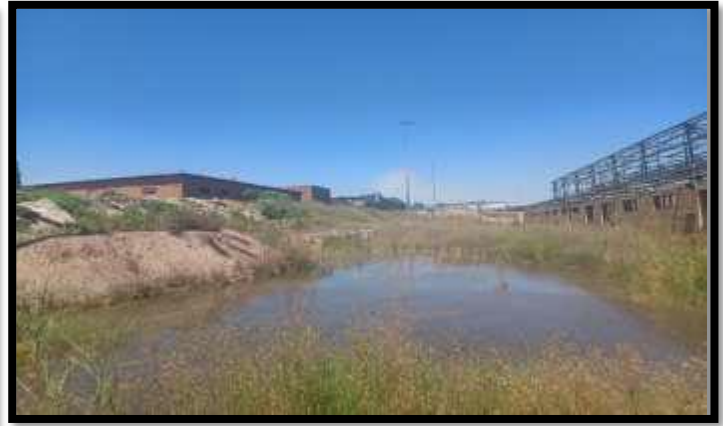
Fig. 2: Stagnant water on site
