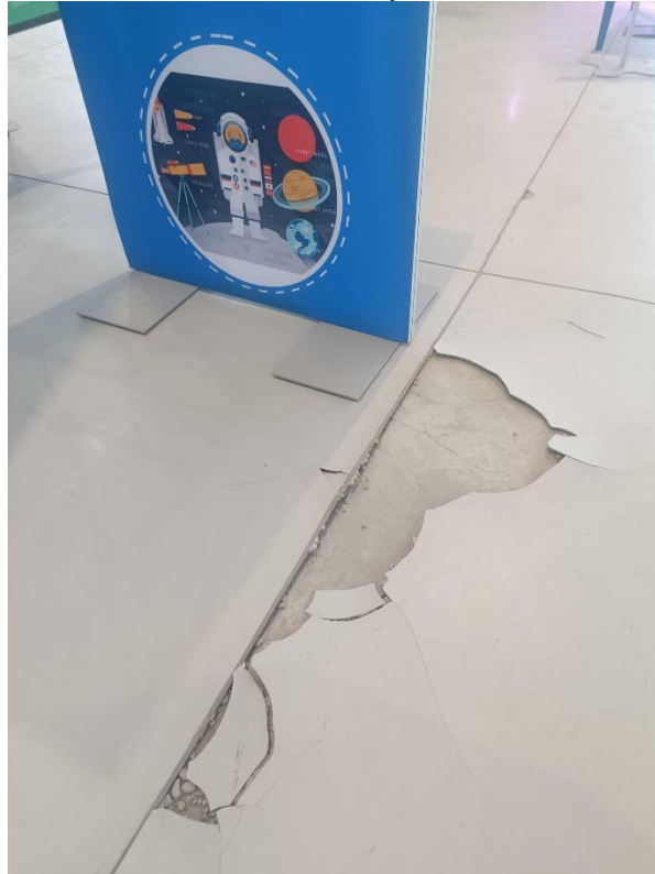
Figure 5. Example of epoxy floor cracks
