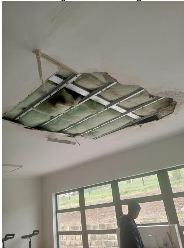
Figure 1. Damage to ceiling due to roof leaks.
