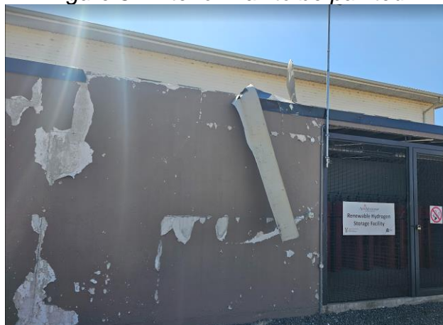
Figure 4. Exterior wall of energy hub to be repainted and flashing to be repaired.
