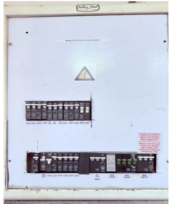
The main 3-phase DB in good condition
