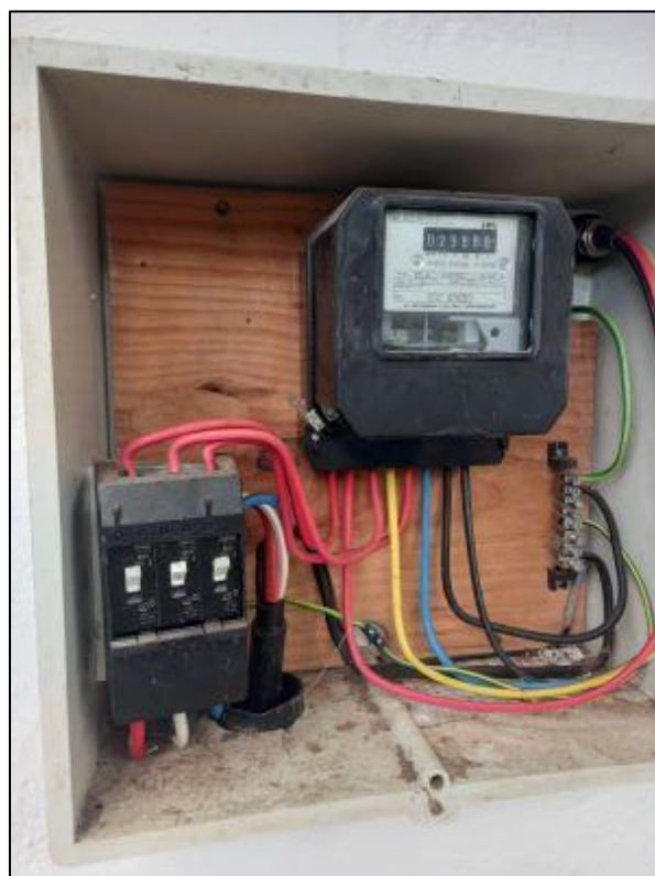
Picture: Municipal meter and 80A 3-phase MCB.
