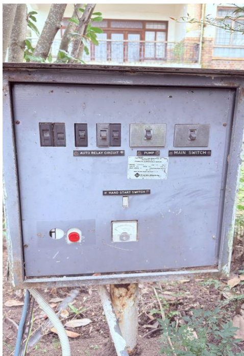
The electrical infrastructure, showing a kiosk and distribution board.
