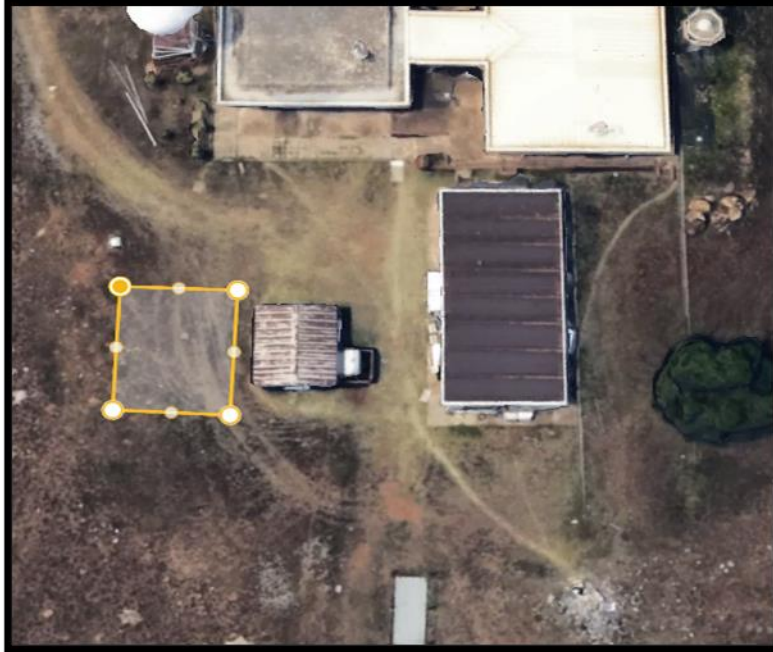
Figure 3 Area that the shelter should be constructed.
