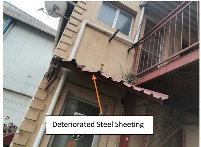
Figure 18: Deteriorated steel sheeting
