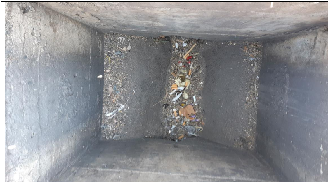
Figure 37 Good condition grid inlet with debris
