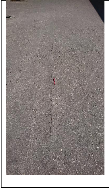
Figure 48: Longitudinal cracks
