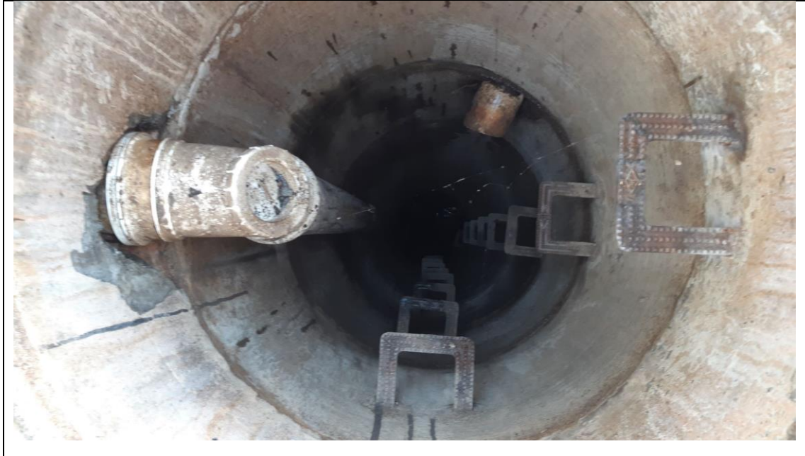
Figure 46 Typical fair condition of sewer manhole. Concrete cracks can be seen around sewer inlet pipe
