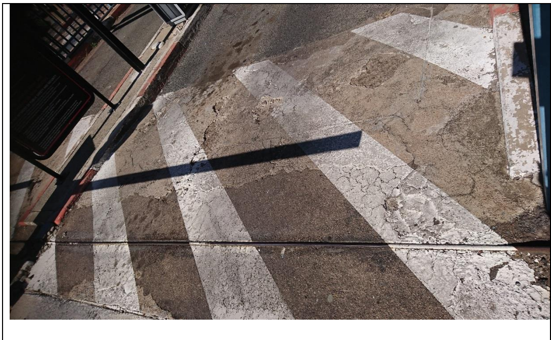
Figure 50: Damaged speed hump
