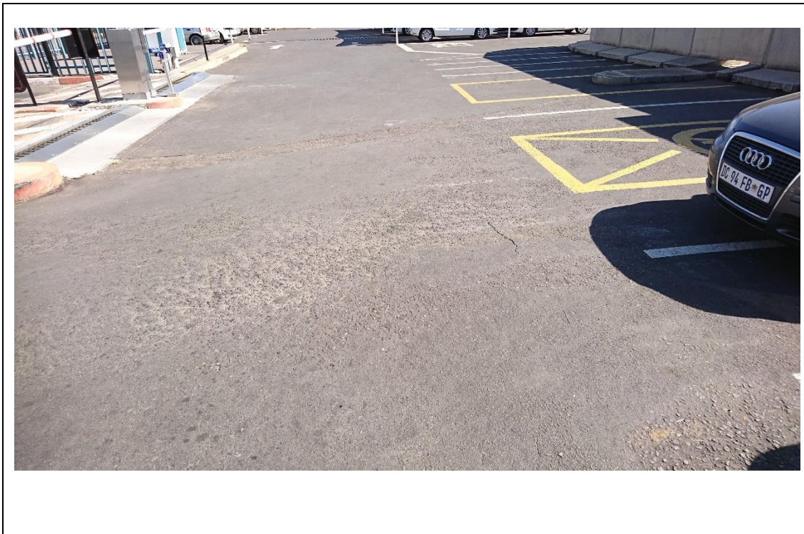
Figure 49: Stone loss at entrance and exits
