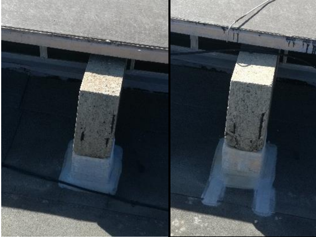
Figure 24 Exposed roof beam reinforcement
