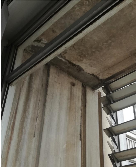
Figure 7 Slab soffit concrete damage
