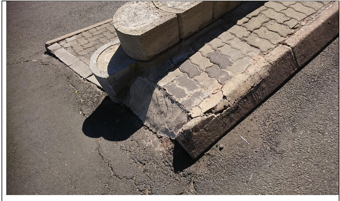
Figure 31 Poor kerb condition
