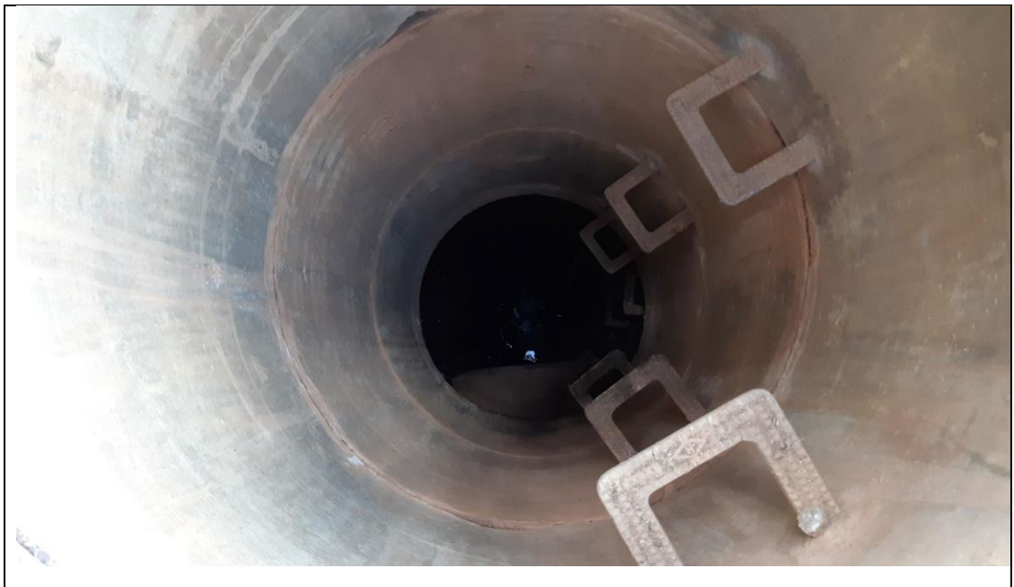
Figure 15 Fair internal manhole condition
