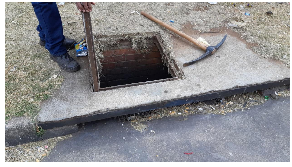
Figure 40 Kerb inlet with narrow opening
