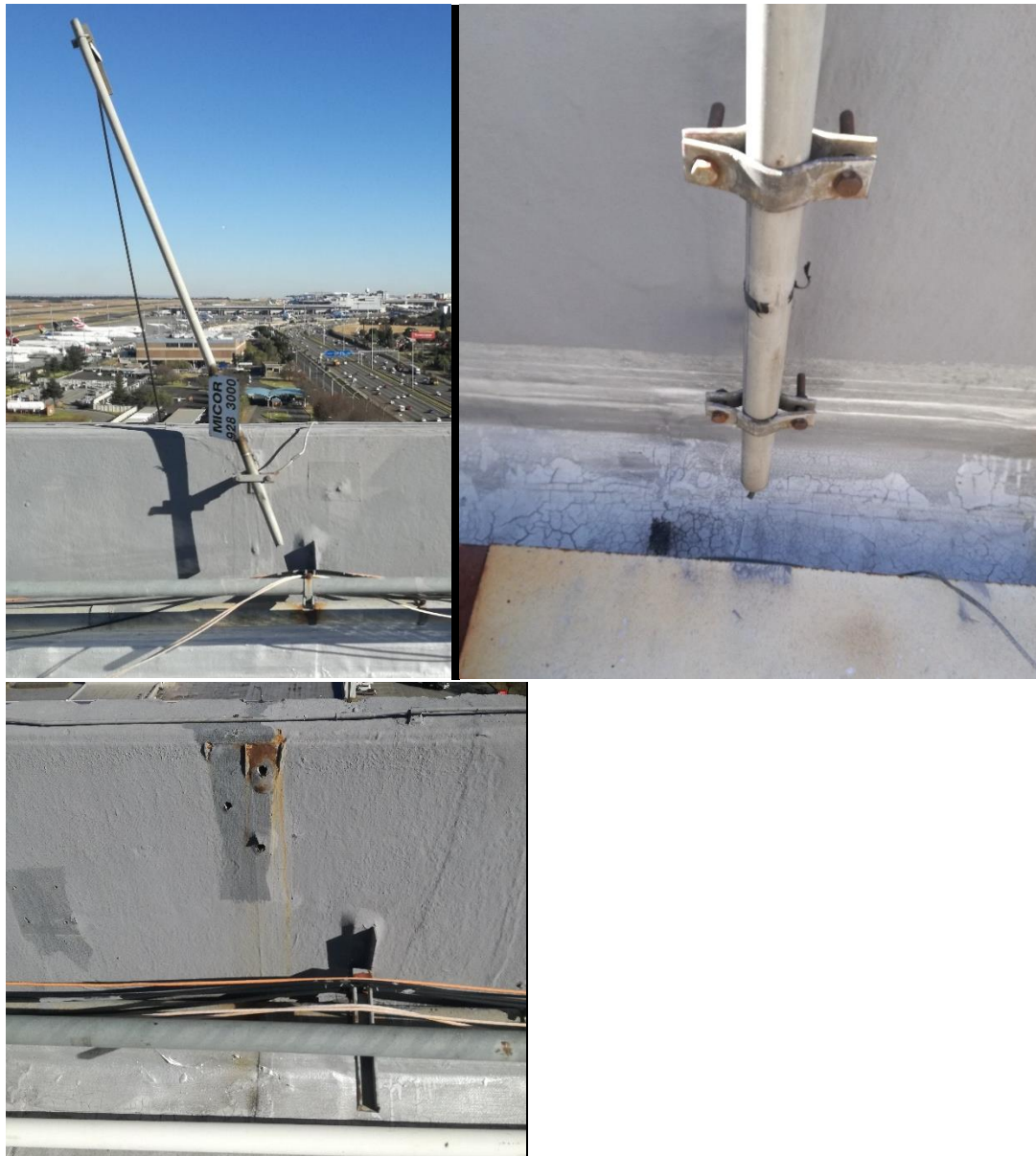
Figure 5 Condition of network masts on roof floor
