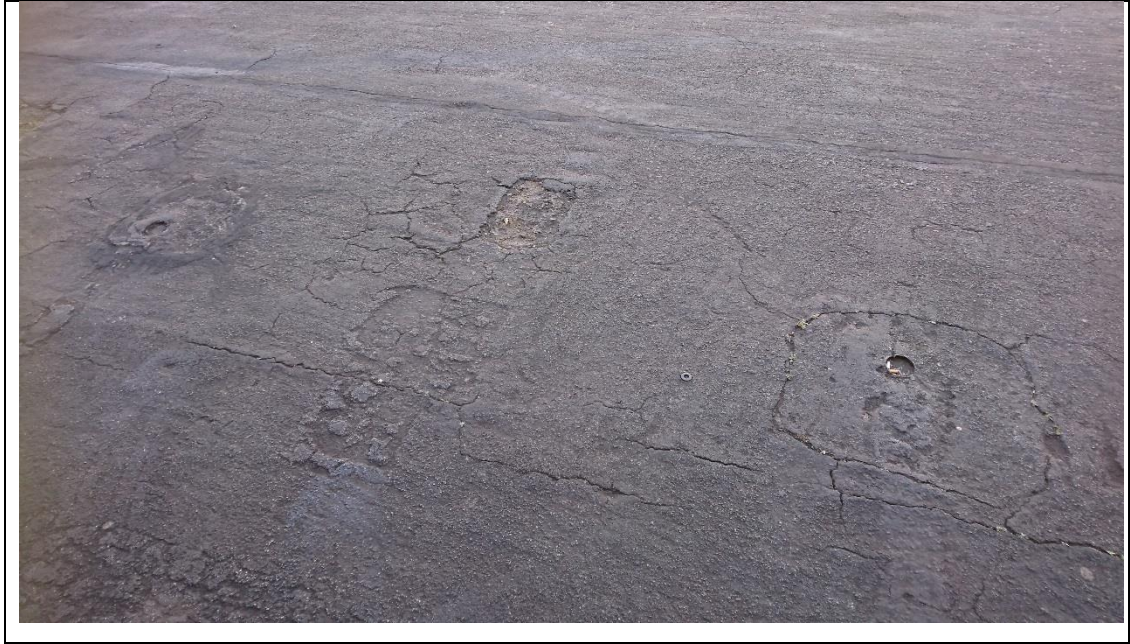
Figure 28 Section pavement failure
