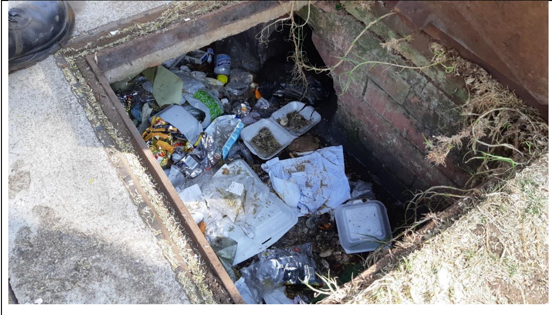
Figure 41 Partially blocked kerb inlet manhole
