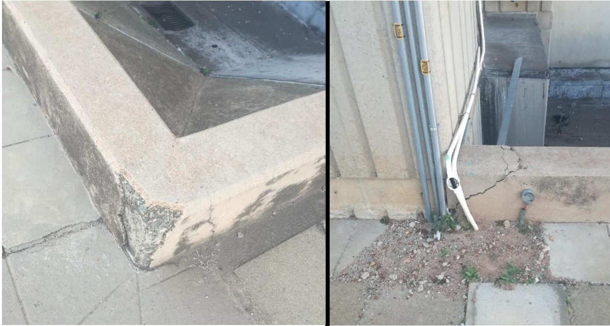
Figure 1 Cracked and exposed concrete walls
