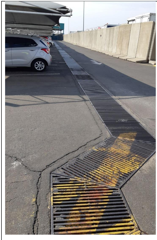
Figure 51 Box drain with grid cover
