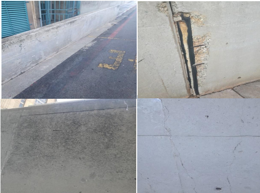
Figure 2 Concrete upstand beam and retaining walls failure
