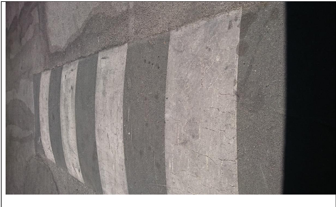
Figure 30 Road marking in poor state, cracked.
