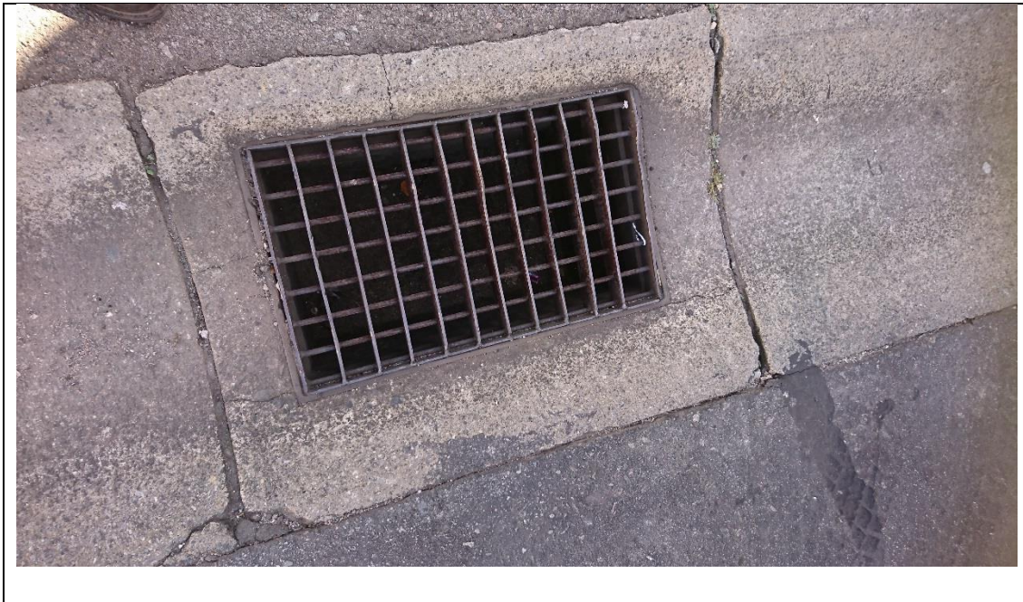
Figure 43: Damaged concrete channel with grid inlet
