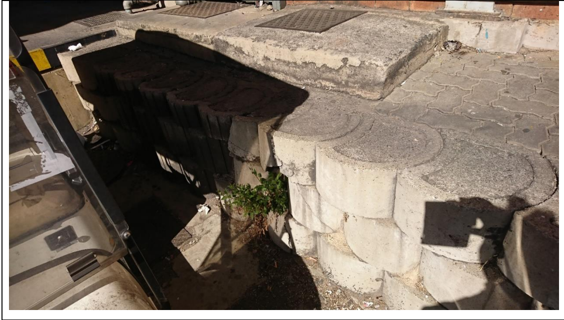
Figure 33 Damaged Loffelstein blocks.
