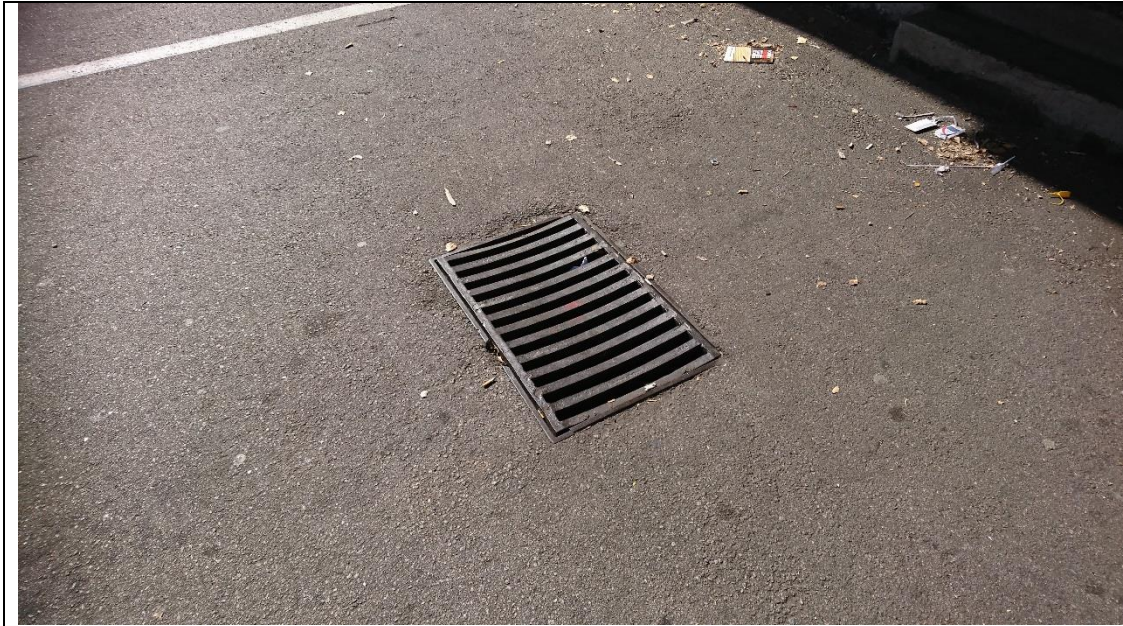
Figure 36 Stormwater Grid Inlet
