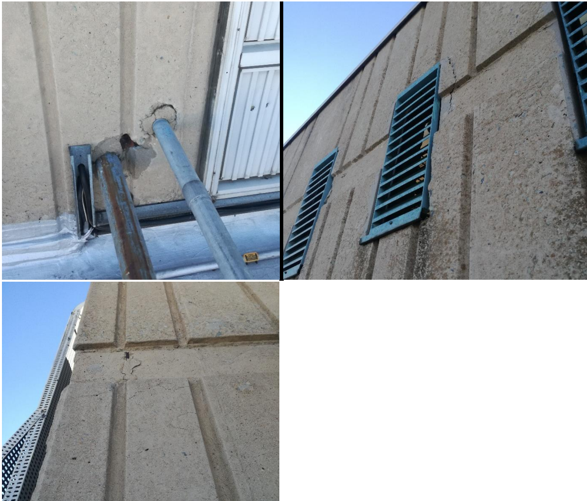
Figure 6 Damaged concrete edges
