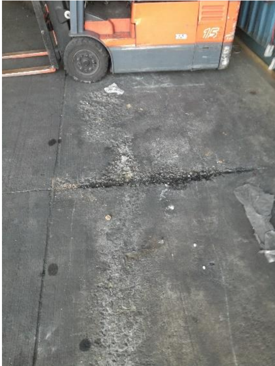
Figure 21 Battery leakage on concrete floor
