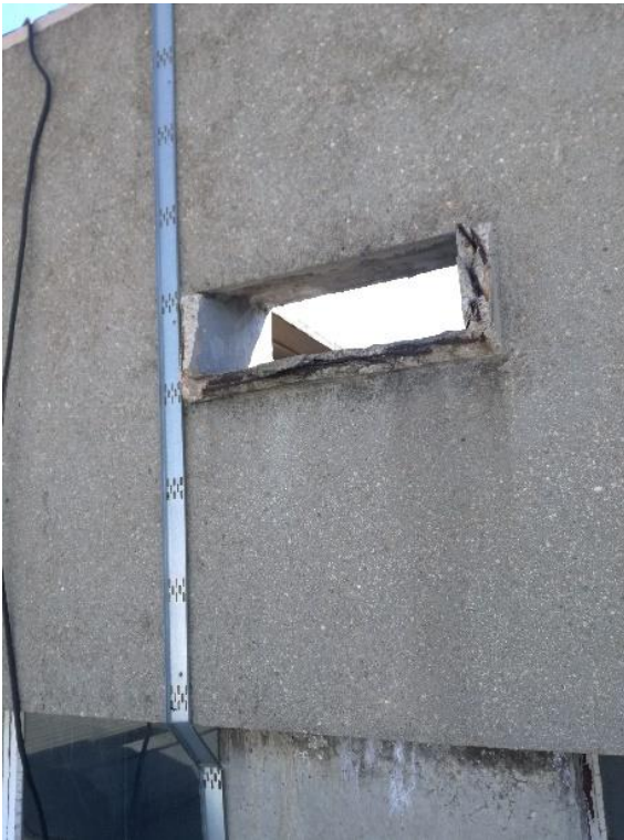
Figure 22 Disintegrated concrete emergency overflow
