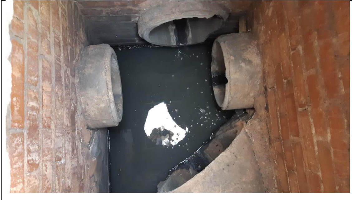
Figure 39 Manhole with stagnant water inside.
