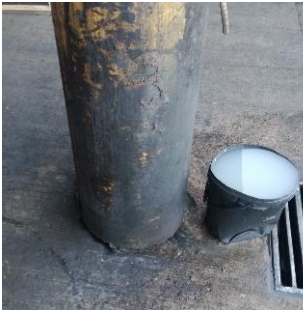
Figure 21 Loose concrete column
