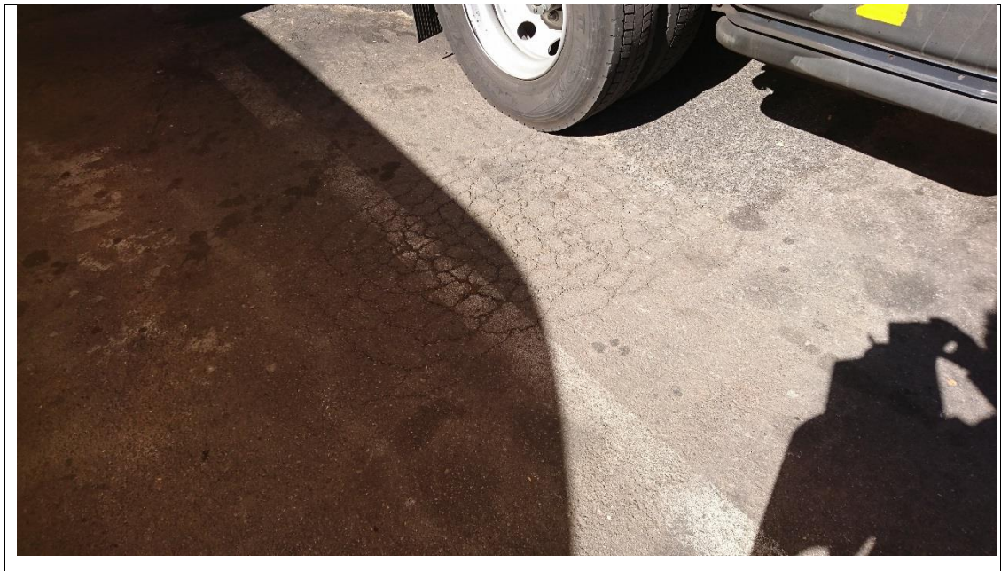
Figure 27 Local pavement failure
