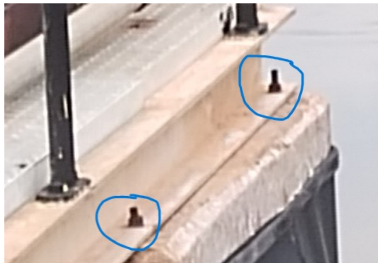
Figure 2: Layout of bolts at the back of the support
