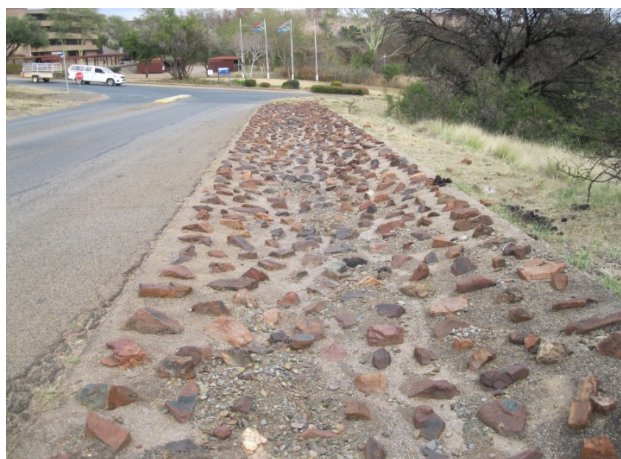
Figure 6: Rocks imbedded in concrete
