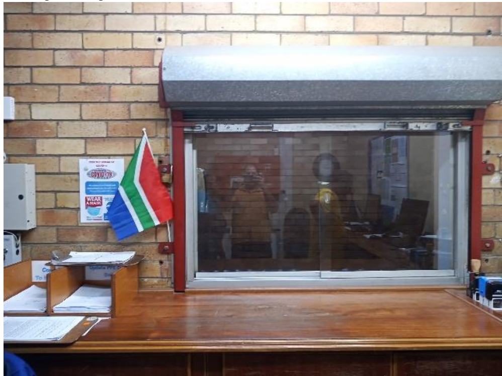
Existing Serving Hatch:
