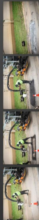
Jetpatcher equipment can be used for repairing many types of asphalt road defects including: potholes, edge breaks, road depressions, wheel path rutting, crack sealing, dig outs, speed bumps, drainage buns, scrubbing
