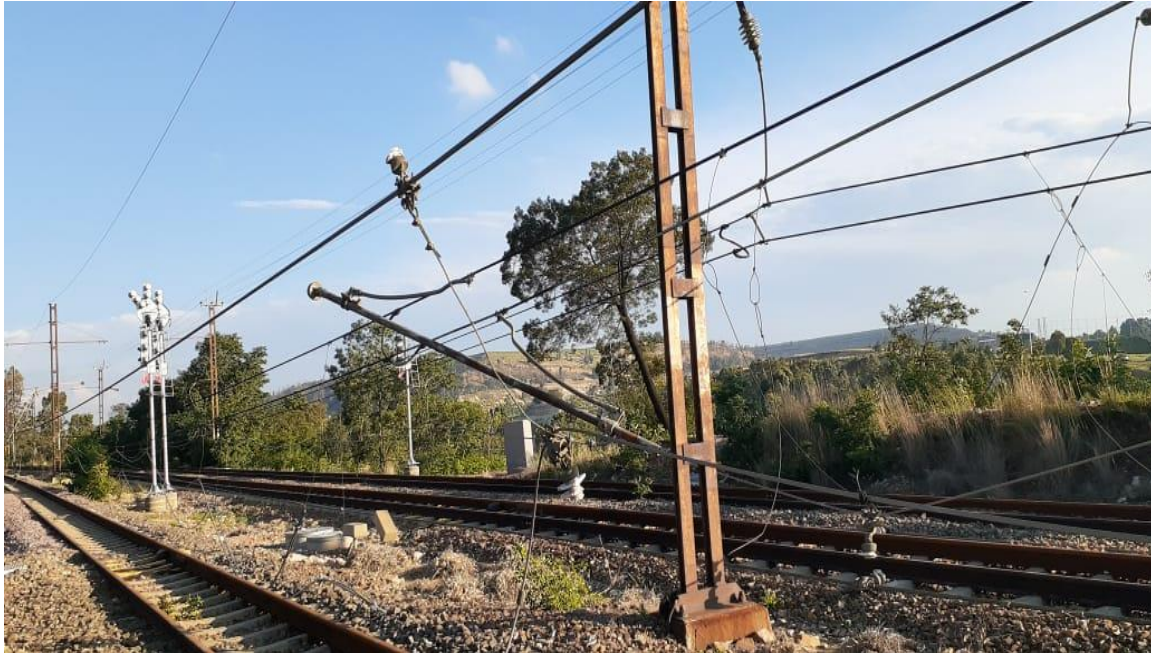
Fig 2.2: Vandalised Track Switch and OHE wires
