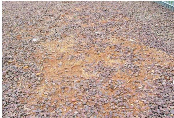
Figure 14: Exposed soil due to poor workmanship
