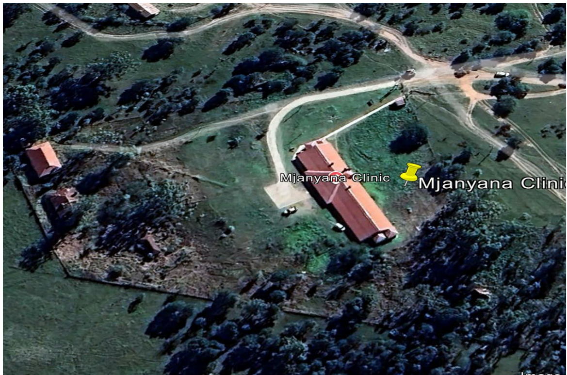
MJANYANA GATEWAY CLINIC AERIAL VIEW (SOURCE GOOGLE EARTH)
