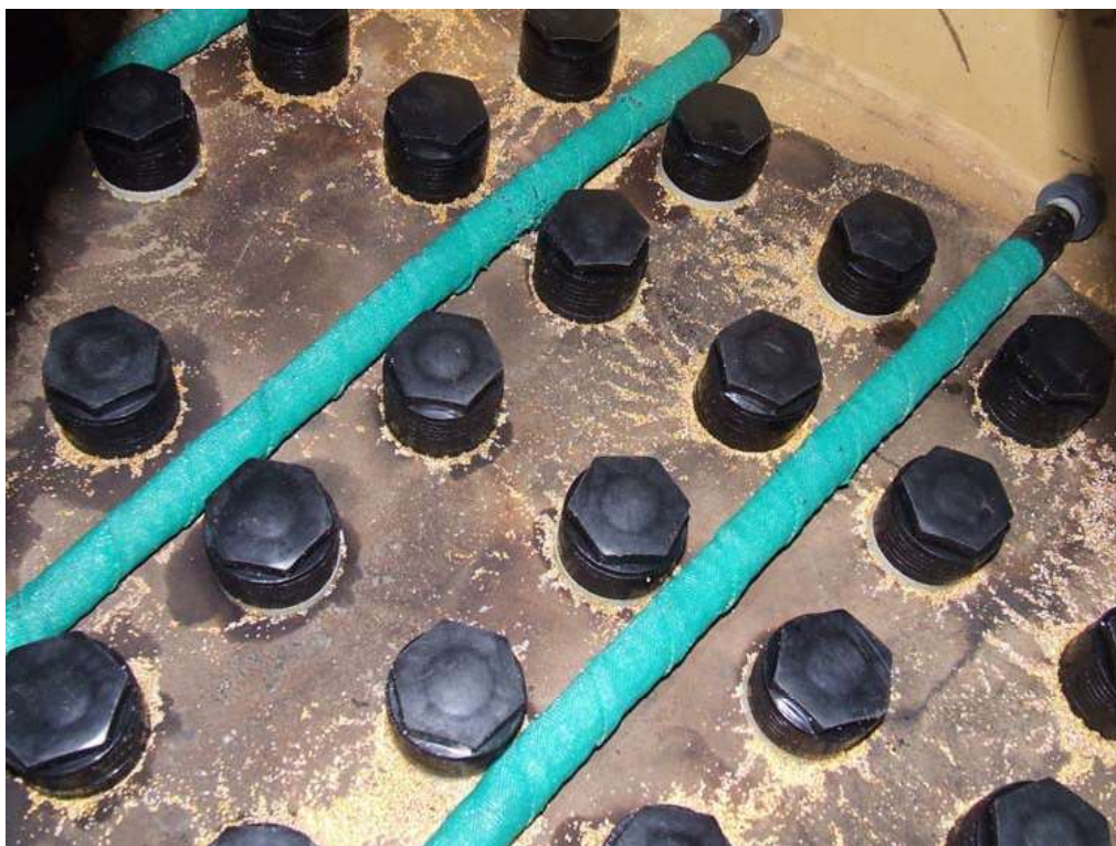
Figure 9: Picture of current mixed bed floor arrangement
