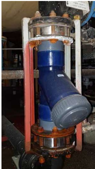
Figure 2: Typical Backwash Outlet U-PVC strainer
