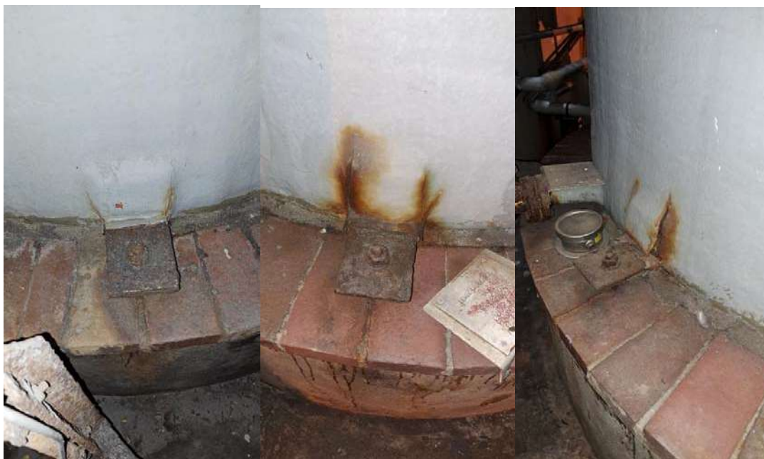
Figure 12: Current Brine measuring tank anchor lugs condition
