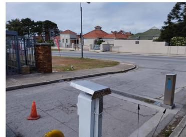
Existing security boom and floor spikes currently unused, no longer functional and redundant due to dirt ingress. Should be removed entirely as position will clash with sliding gate.
