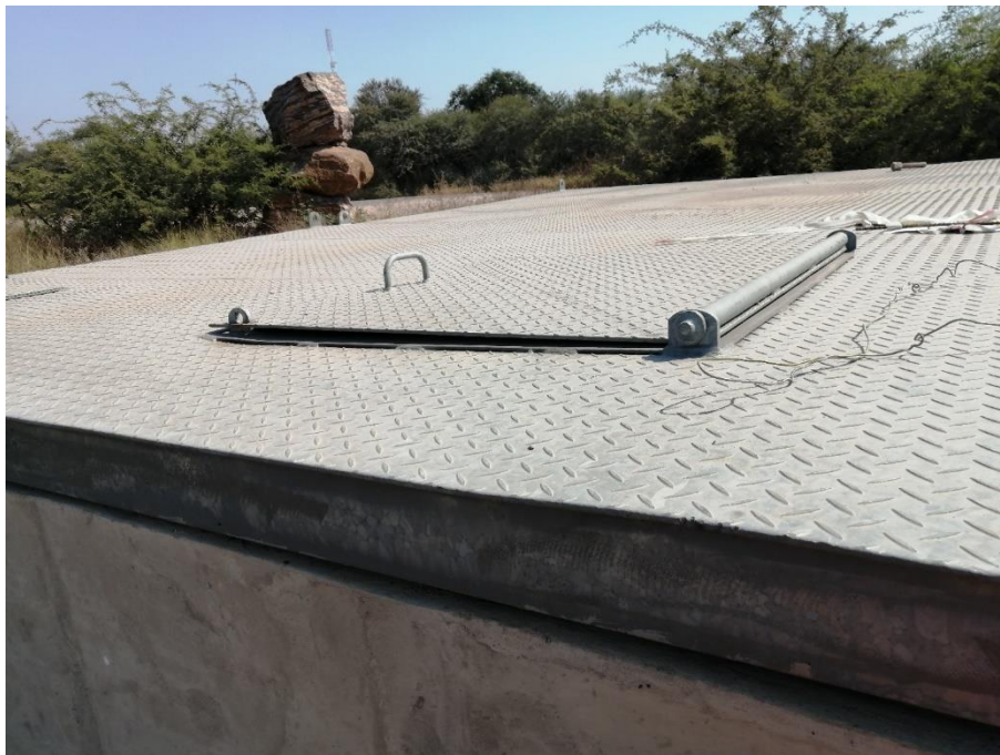
Figure 3: Chequered plate covering and hatches on the valve pits that require security locks to be added to prevent unauthorized access.
