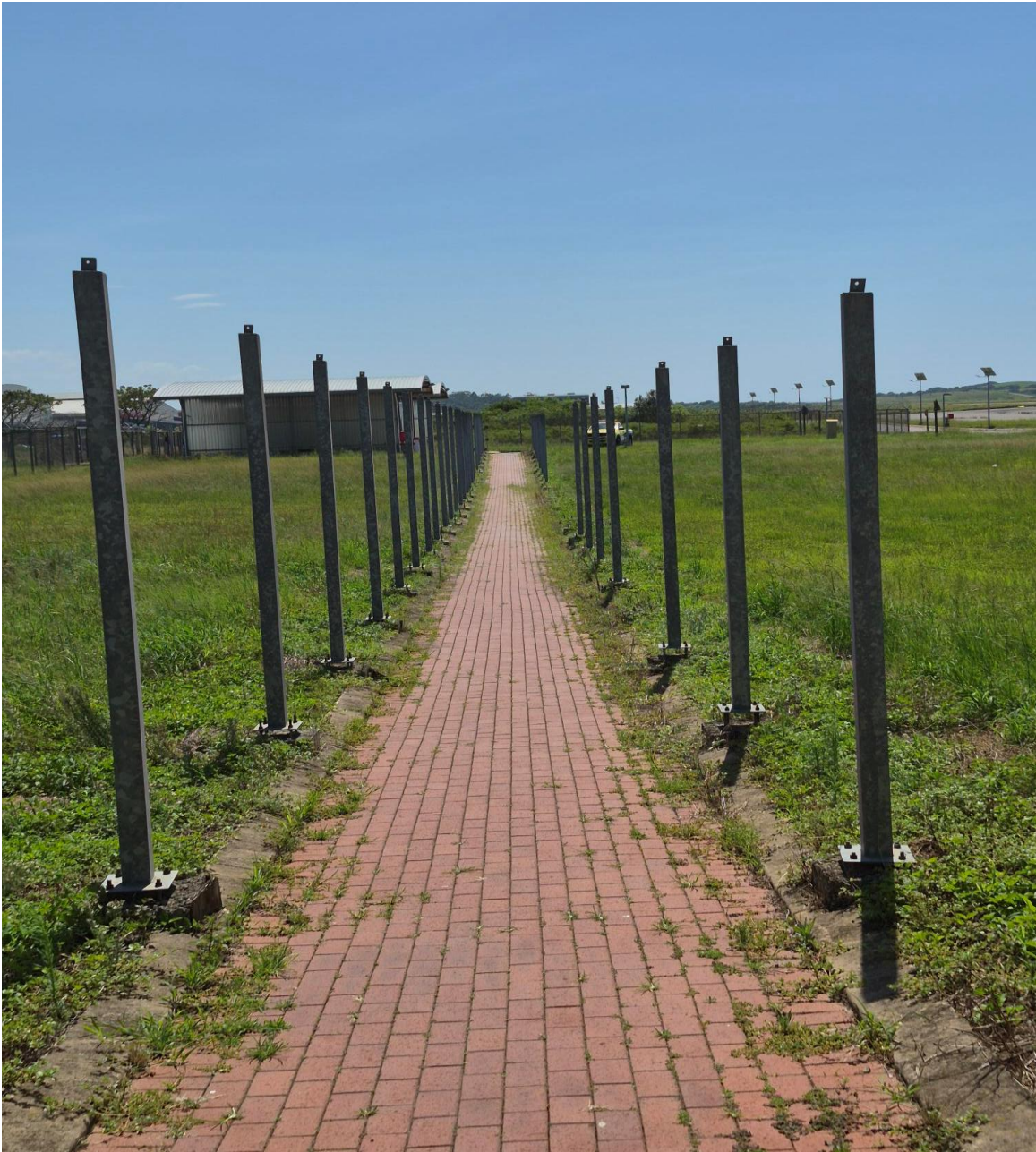
Existing Paraplegic Ramp:
