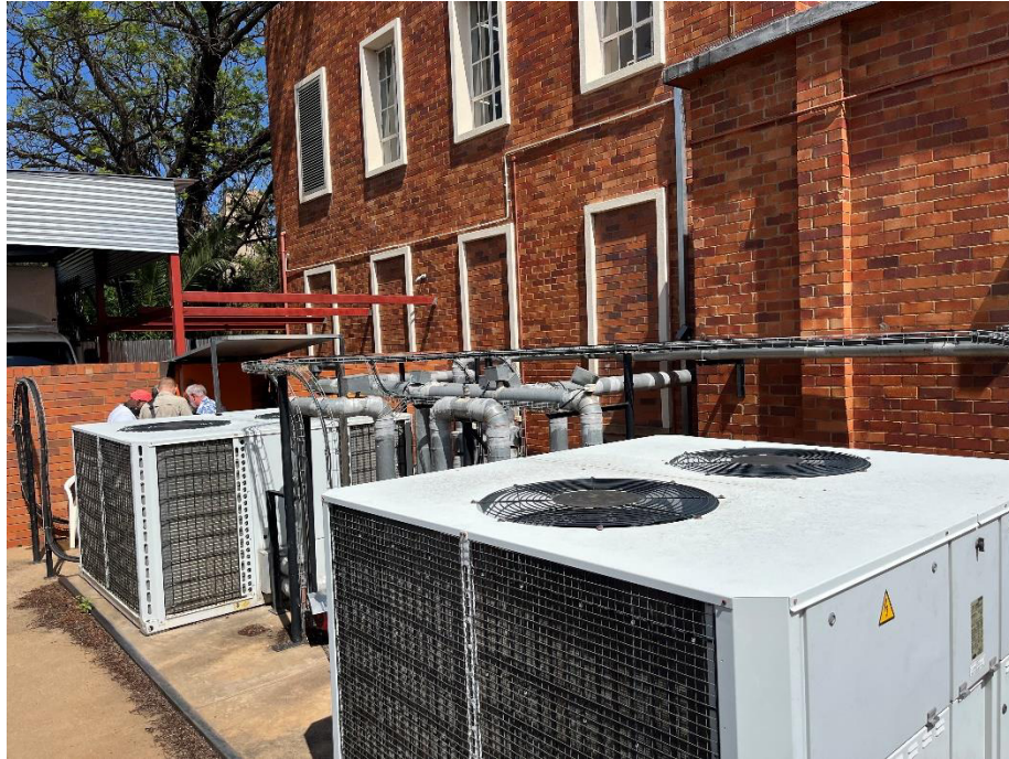
The existing chiller and chilled water pumps.
