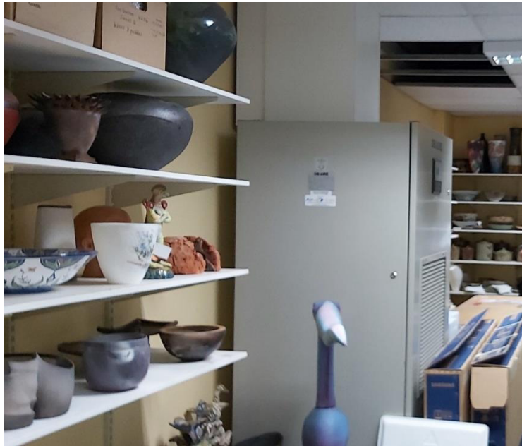
The existing closed control Dunham bush DX split unit.
