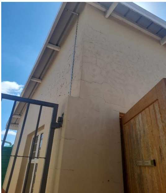
Fig 3: Paint to walls
