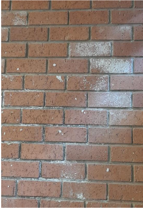
Fig 17: High pressure cleaning
