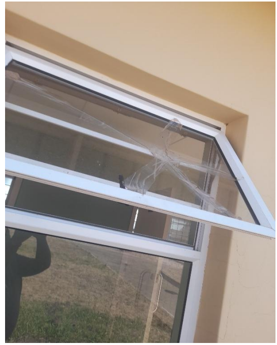
Fig 10: Replace glazing
