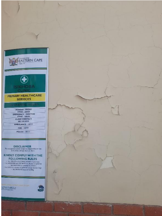
Fig 1: Peeling paint
