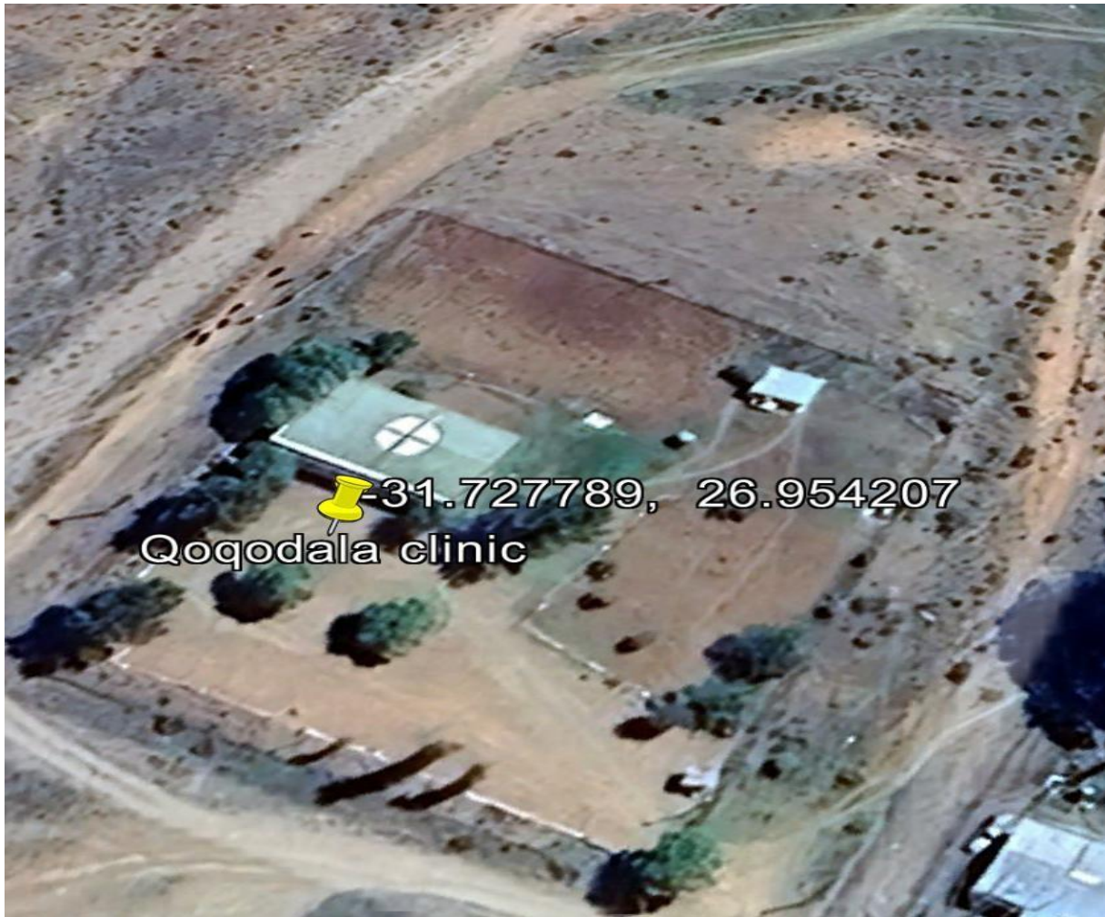
QOQODALA CLINIC AERIAL VIEW (SOURCE GOOGLE EARTH)
