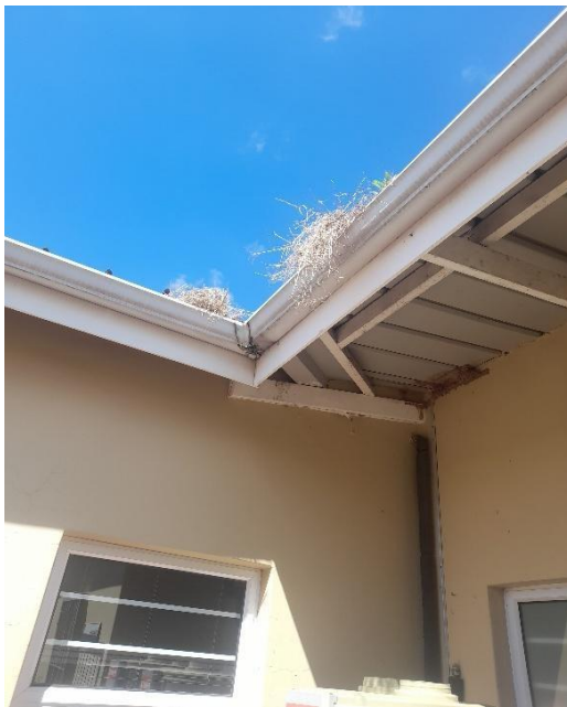
Fig 7: Cleaning of gutters
