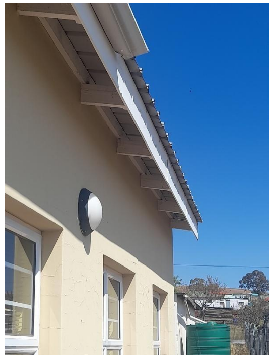
Fig 12: Replace damaged gutters
