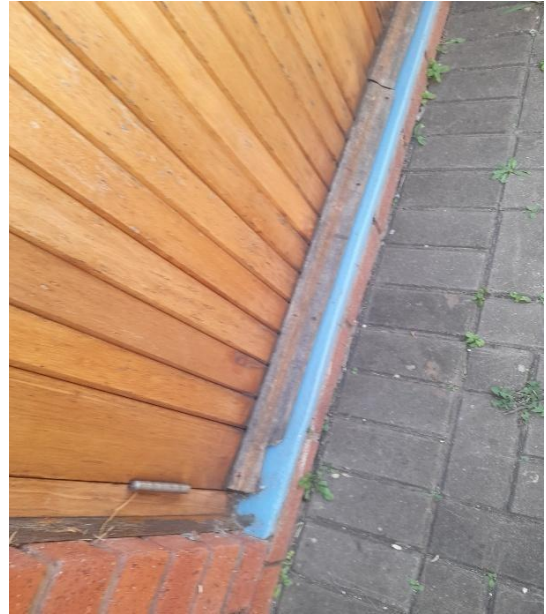
Fig 6: Replace weatherboards
