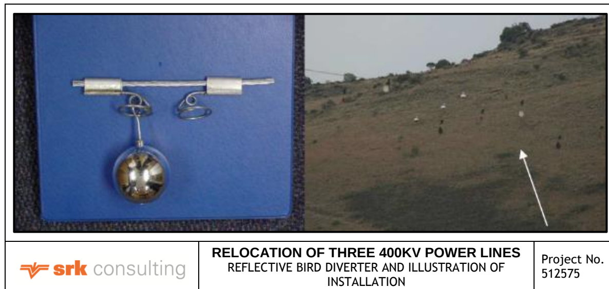
Figure 5-19: Reflective bird diverter is represented on the left and on the right is an illustration of it installed with conventional bird flapper (van Rooyen, 2009).
