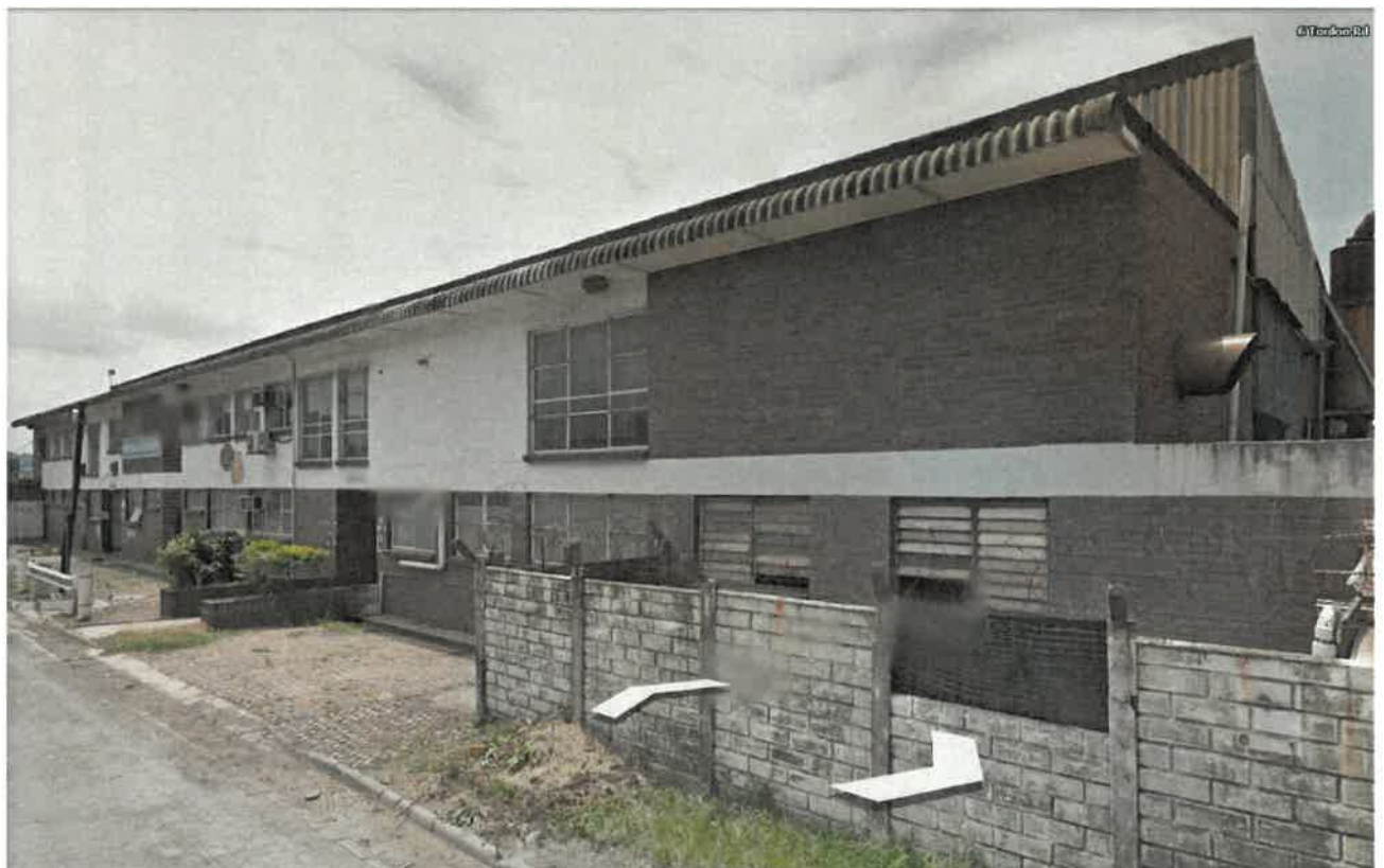
06 Toulon Road Building front view
