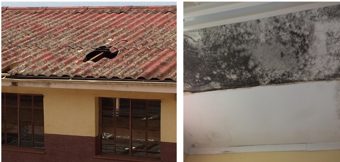
Roof Sheeting and purlin blown off and trusses damaged
