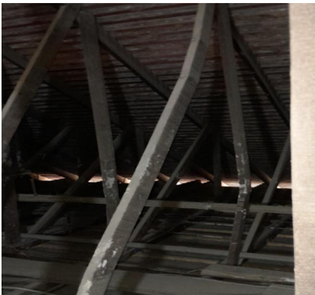
Figure 4 and 5: Showing damaged web members
