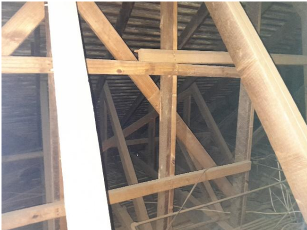
Figure 8 and 9: Showing laminated member in the roof
