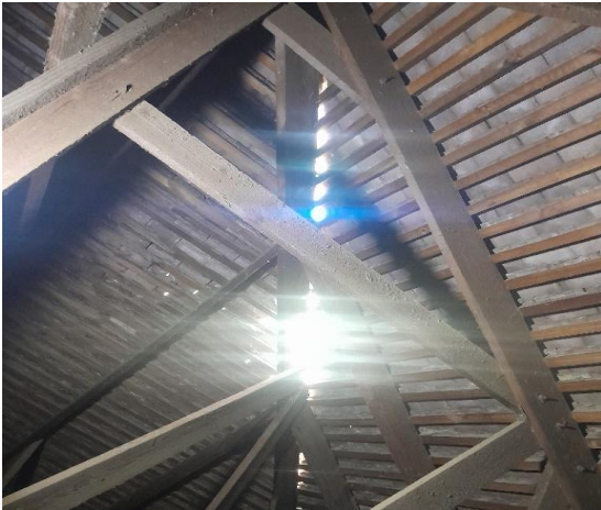
Figure 6 and 7: Showing damages on the Hip rafter and damaged roof tiles
