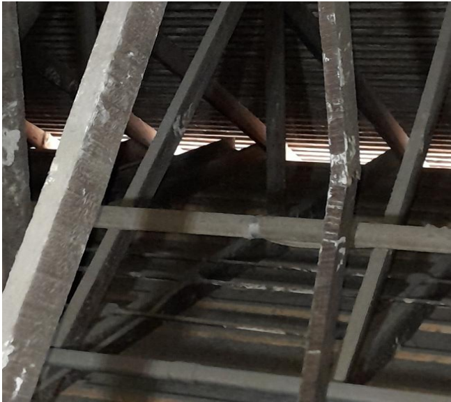
Figure 2 and 3: Showing Web member of the truss that are damaged
