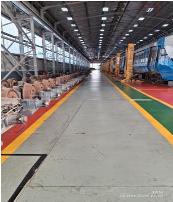
Lifting Shop & Rolling Stock Train Pits
