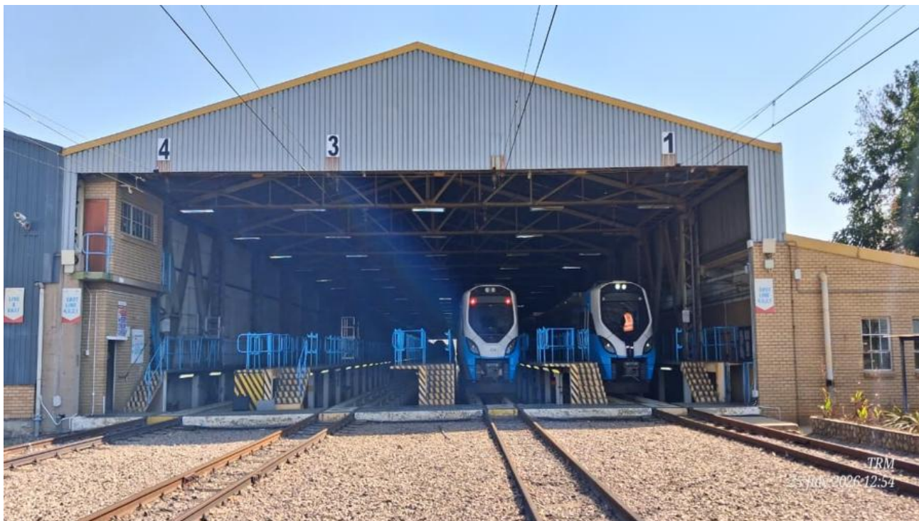
Figure 1 Gibela & Rollingstock Maintenance Sheds
