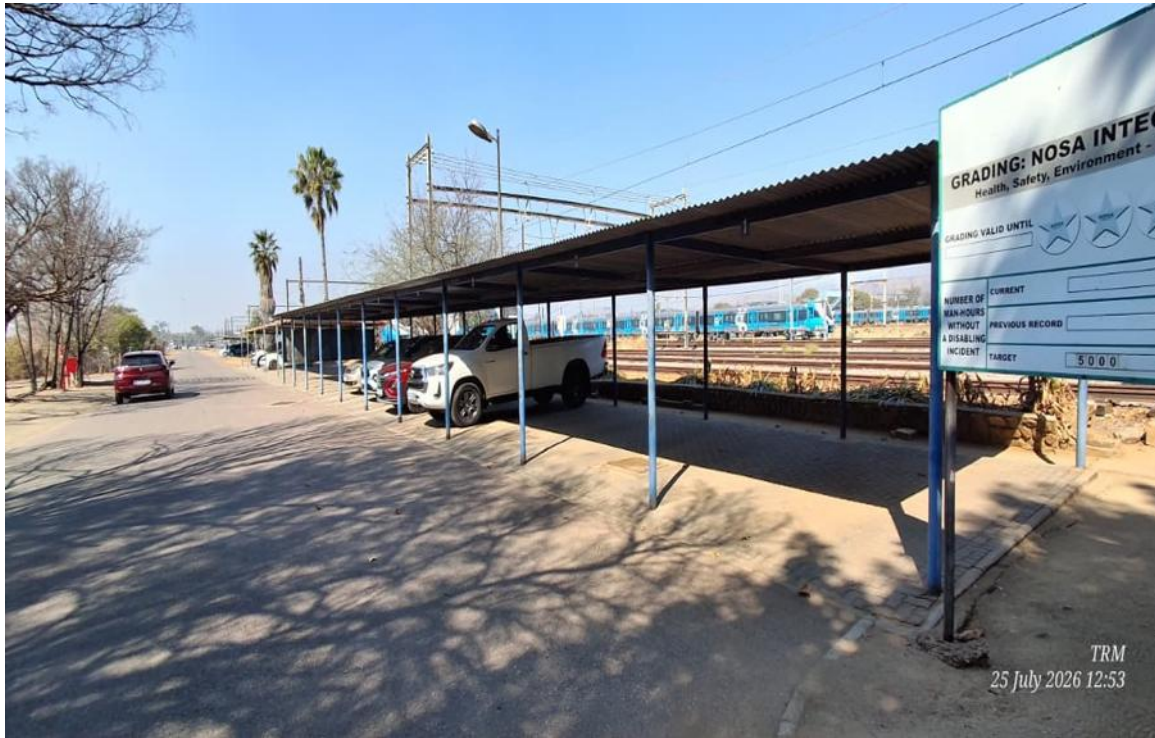
Parking Bays with paving & Tar road
