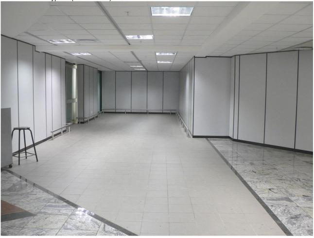
This type of internal hoarding will be applicable where construction work takes place adjacent to other tenants to minimise noise, dust and visual screening.
