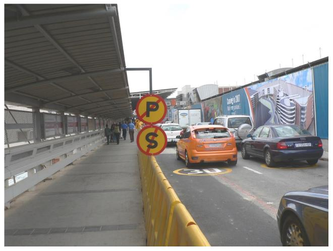
Yellow New Jersey barriers or orange plastic netting (at the discretion of the KSIA-Project Manager) must be used to barricade the construction site from the public prior to construction work taking place.
