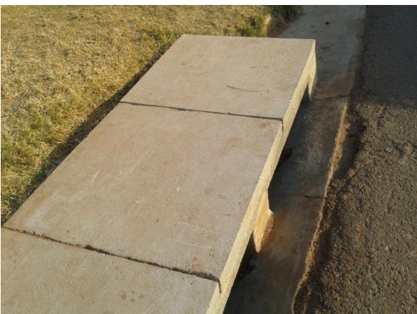
220 x 220 brickwork, plastered, 2-3 courses @ 1.5m-1.8m spacing
