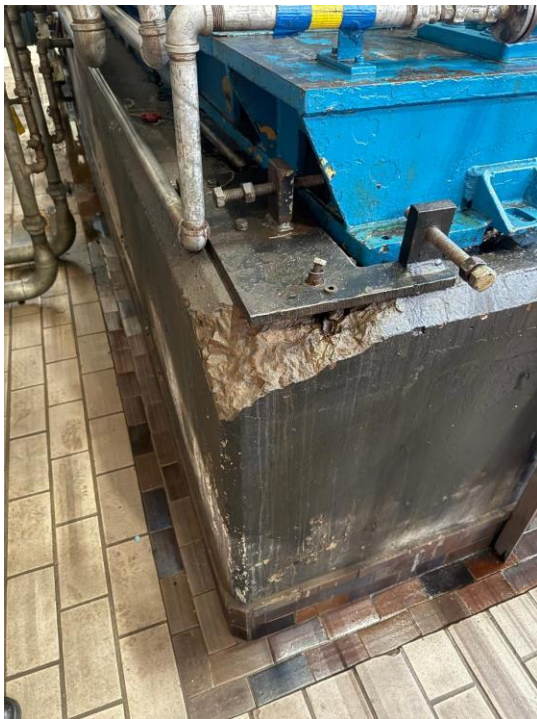
Figure 1: Spalled Concrete and Dislodged Anchor Bolt
