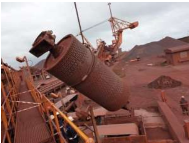
Picture 1: Pulley replacement
