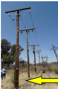
Pole Number BD1 Termination point – Start dismantling from this pole
