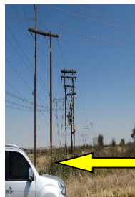
Pole Number BD56 – End dismantling at this point
