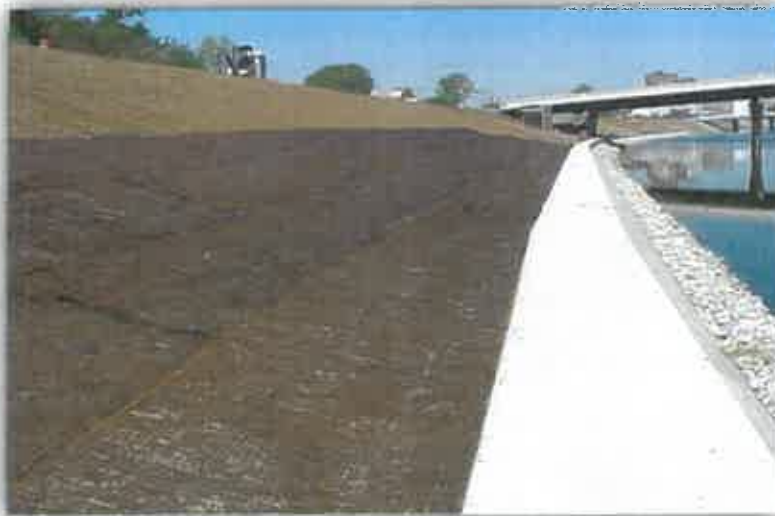
Figure 2 Geo-fabric installed and pegged down on a slope to retard soil erosion. Vegetation may grow threw the blanket over time.
