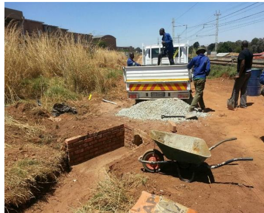
Installation of stormwater pipes
