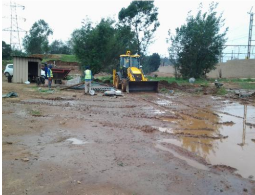
Tlb open earth drainage at Geldenhuis
