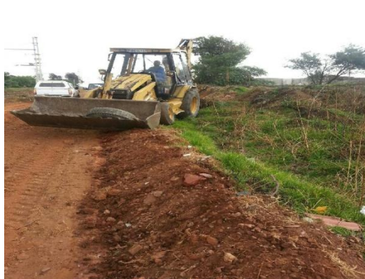
Tlb open service road and drain at Princess
