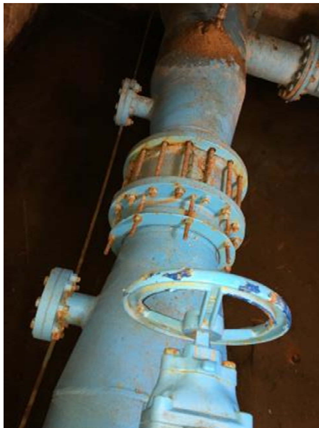
Non-return valve installation at Bospoort WTP
