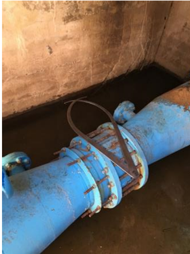
Non-return valve installation at Bospoort WTP
