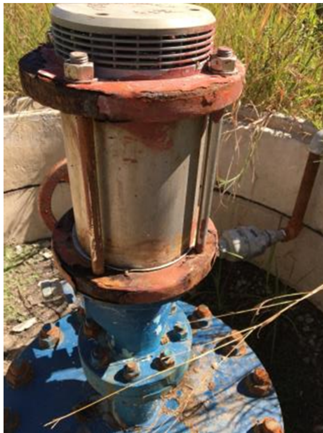
First air valve from Bospoort WTP
