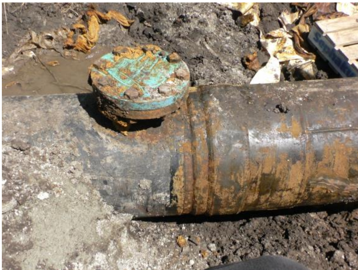
Excavation at leak site. Sintakote (left), petrolatum tape wrapping (right). No pitting.
