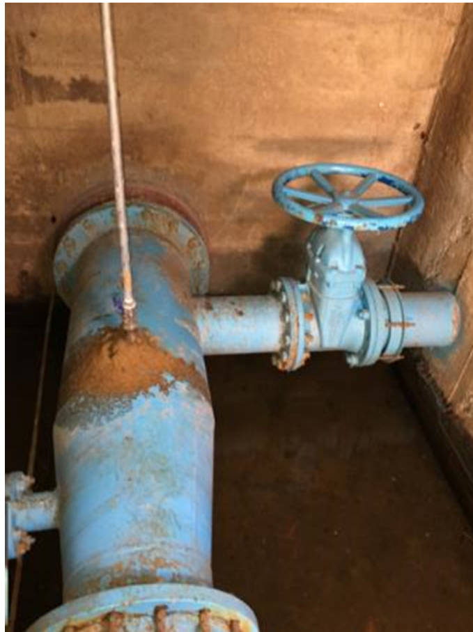
Non-return valve installation at Bospoort WTP
