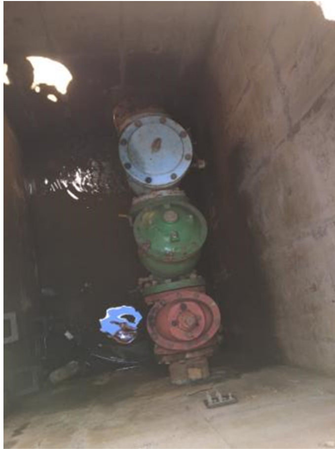
Old cross-connection between Bospoort pipeline and Magalies Water Vaalkop pipeline
