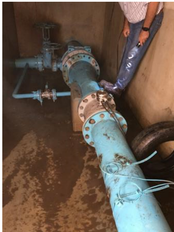
Water meter and scour installation downstream of Bospoort WTP high lift pumping station
