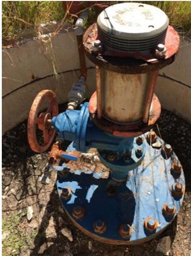
First air valve from Bospoort WTP
