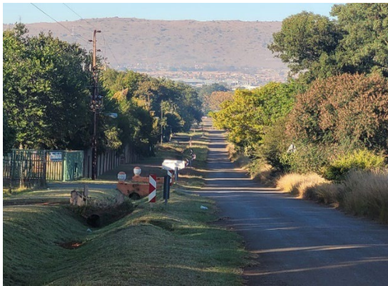
Photo 1 – Renet Avenue (Eastern Boundary of Site / Study Area)
