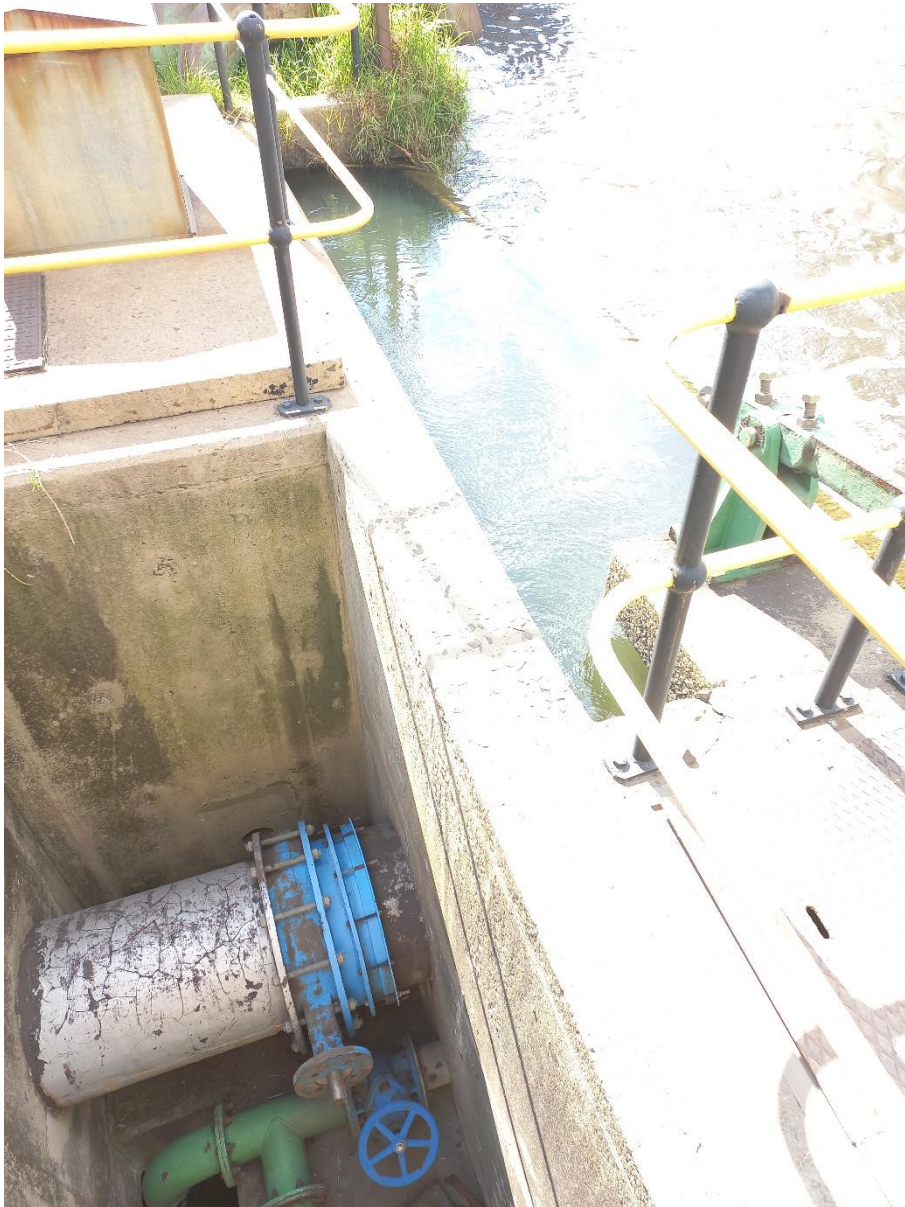
Supply pipe protruding the wall (RH) to the float valve
