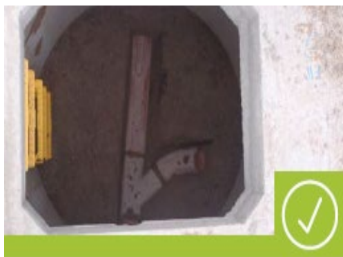
Example of a manhole benching
