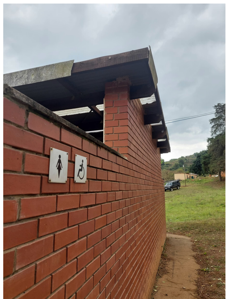
Figures 3 & 4: Exterior images of the staff ablutions (left) and boys' ablution (up) showing damaged fascia and barge boards, as well as missing downpipes
