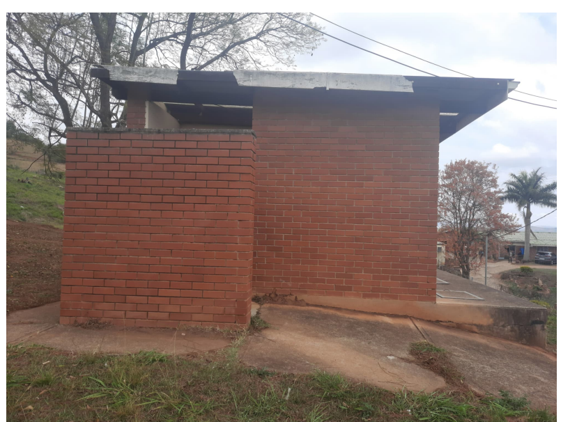
Figures 3 & 4: Exterior images of the staff ablutions (left) and boys' ablution (up) showing damaged fascia and barge boards, as well as missing downpipes
